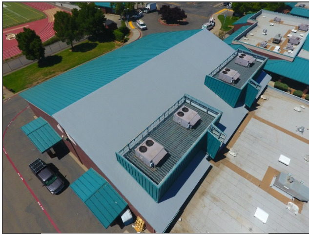
New gym roof at Sheldon High School
