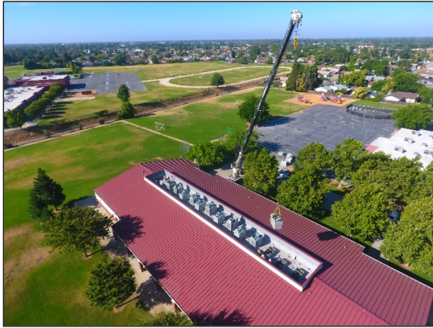
Installation of new rooftop HVAC units at David Reese Elementary
