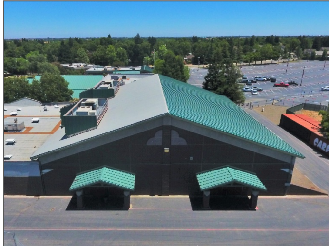
New gym roof at Laguna Creek High School
