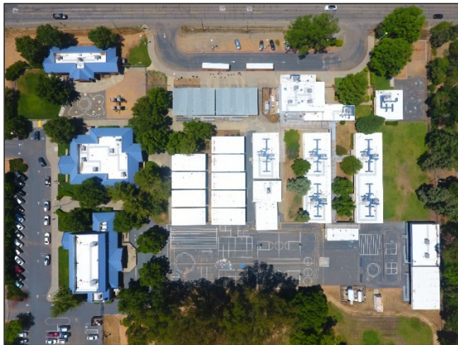
New roofing campus wide at Sierra Enterprise Elementary
