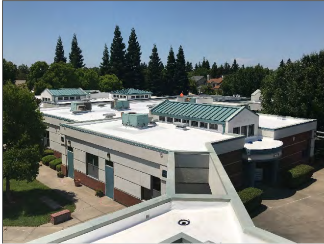
New Roofing at Barbara C. Morse Elementary School
