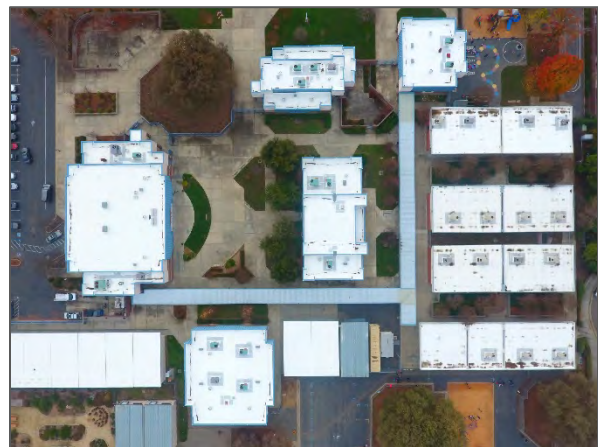
New roofs at Foulks Ranch Elementary School
