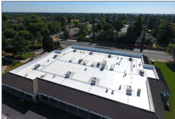
New HVAC Units at Elk Grove High School
