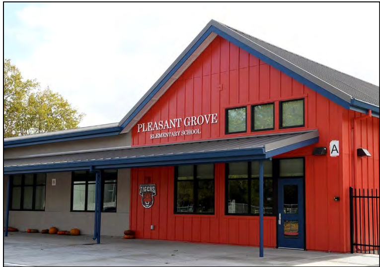
New administration building at Pleasant Grove Elementary School.
