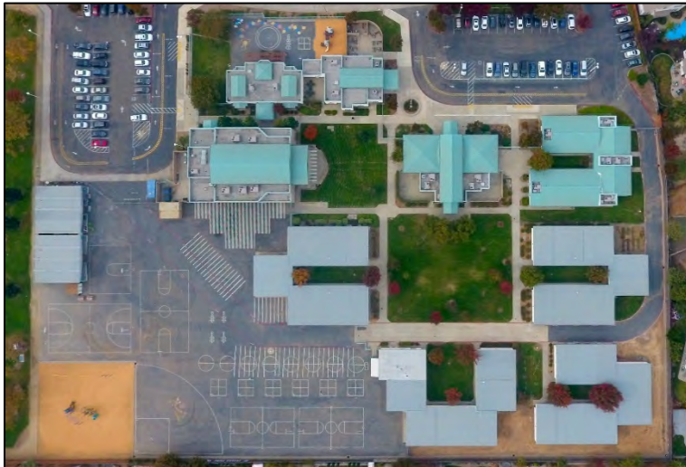
New roofing at Case Elementary School
