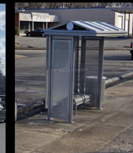
Bus shelter at Park Ave
