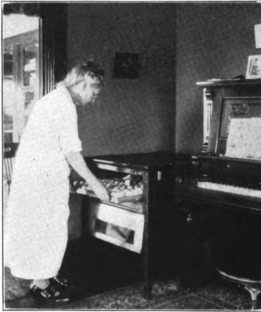
Figure 8. Electric incubators are easily controlled, provide a very uniform heat, and require little attention. Freedom from odors permits of their operation in the house. The incubator shown is located on a LaPorte County farm and hatched 66.9 per cent of the eggs the first time it was operated (April, 1926). Tests on this and other 150 egg machines show a consumption of 22 to 30 K. W. H. per hatching period, costing from .88 to $1.20.
