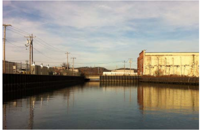
Existing bulkhead along the Mill River
