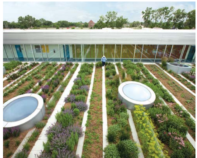
Rooftop urban farm, Chicago, IL
