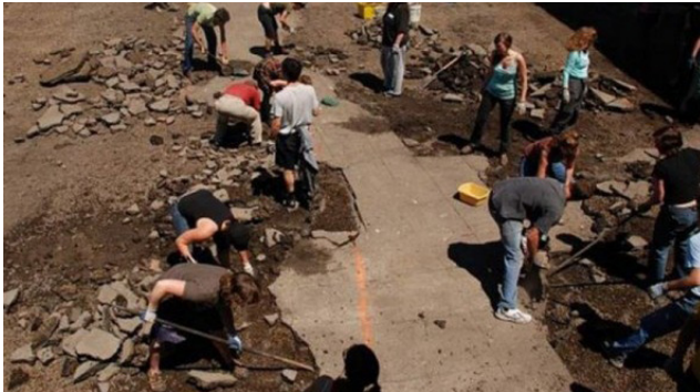
Depaving (top row): The Fargo Forest Garden in Portland Oregon, replaced 3,000 square feet of asphalt with a community garden.
