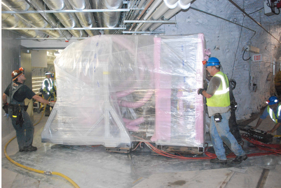
Figure 2.10. The LUX Detector arriving underground and being pushed on the air skate system. Compressed air, carried in the yellow tube to the control panel, visible on the right of the photograph, pushed down from seven "air skates" that LUX rested on. This caused the transport unit to hover, and it could be pushed, providing the maneuverability necessary to negotiate the tight underground tunnels. The sheet metal visible on the ground provided a smooth, continuous surface for the air to push against. Photograph by Matt Kapust.
