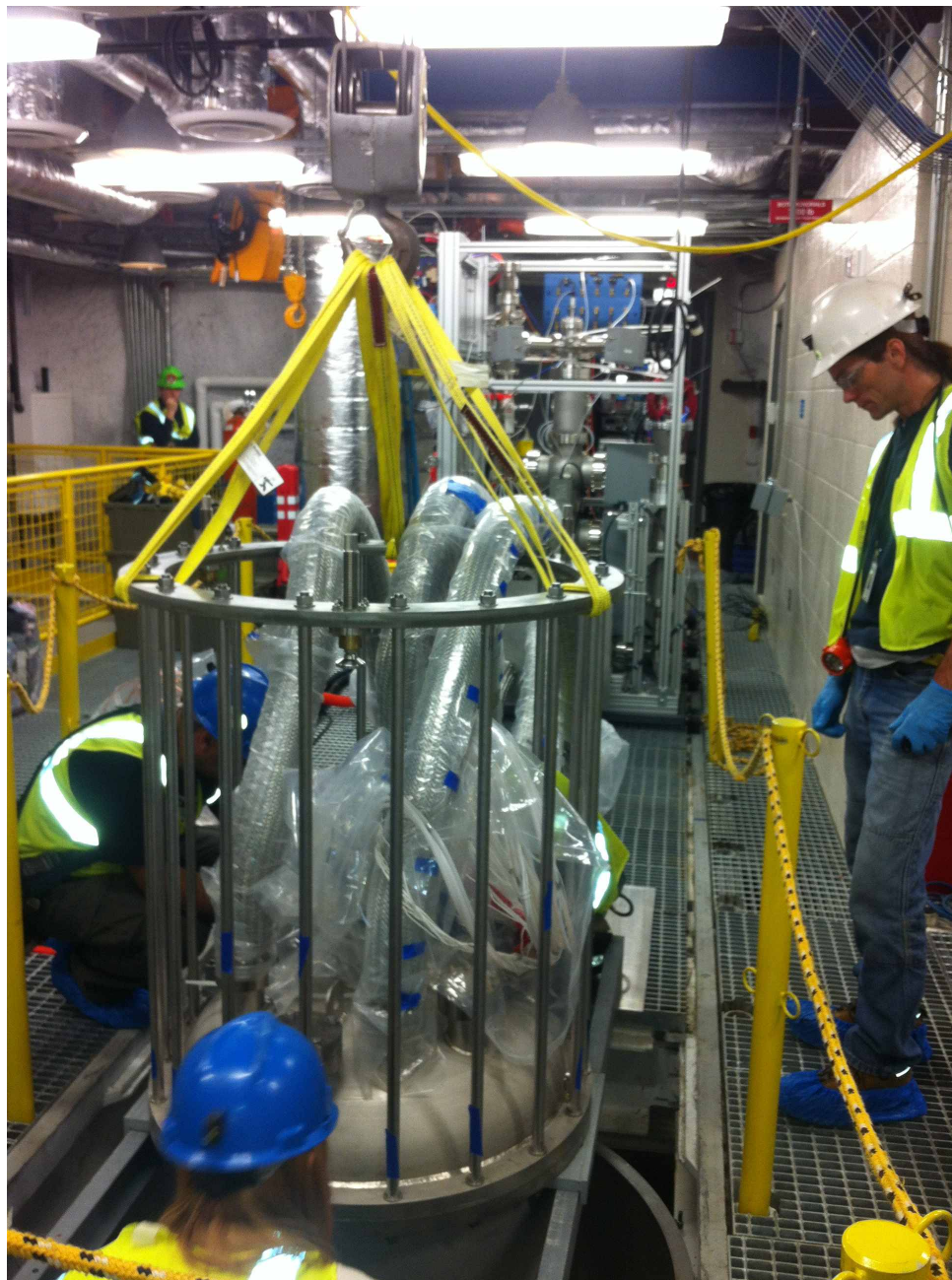
Figure 2.11. Due to overhead clearance constraints, the detector needed to be lowered into the tank in three stages. After each stage, additional infrastructure was built above. Here, the support ring is being installed. The detector hangs one meter below the support ring, and all other infrastructure is mounted above it. This minimizes the material close to the detector. Photograph by Jeremy Mock.
