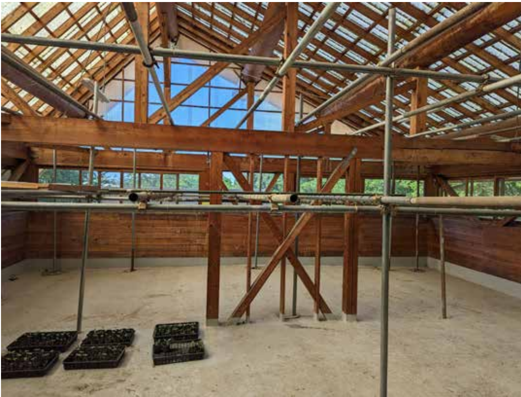
The Farm Shop's upper level shows off sustainable design features, including an exposed timber structure, ample daylighting, and natural ventilation.
