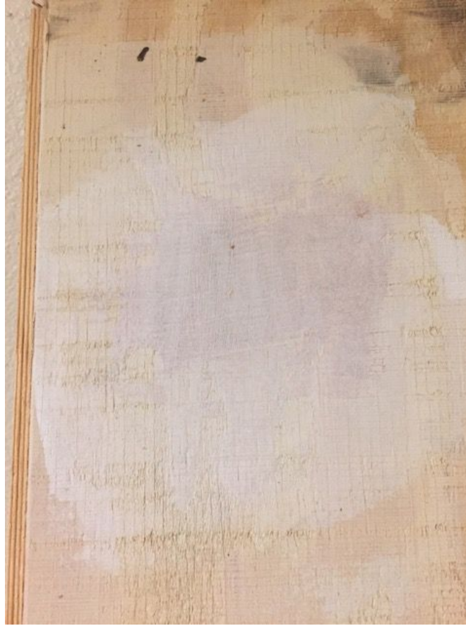
Figure 1.6: HPM provided a mockup of the exterior wood siding post-installation. HPM includes patching for insulation holes in their installation process, though the Gardens plans to employ its own staff for painting.
