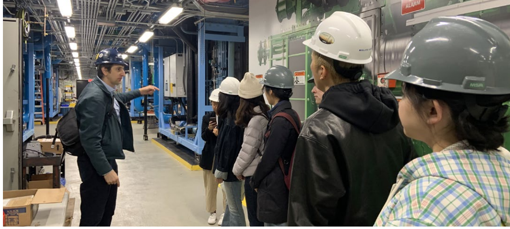
Urban Tech students visit Hudson Yards to learn about innovative approaches to energy production and management in the development's cogeneration plant.
