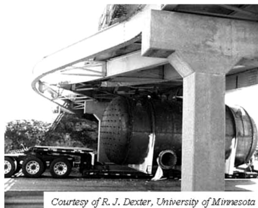
Fig. 1 Example of catastrophic bridge damage due to a vehicular impact
