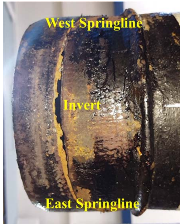
Figure 3.20. Damage at TR Flex® Plain End after McWane SFC Bending Test 1 (3-9)
