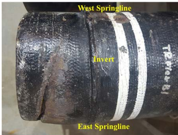
a) View from Invert
