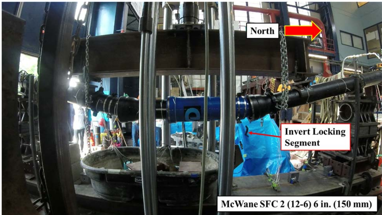
Figure 3.25. Invert Locking Segment Fell out of P Joint
