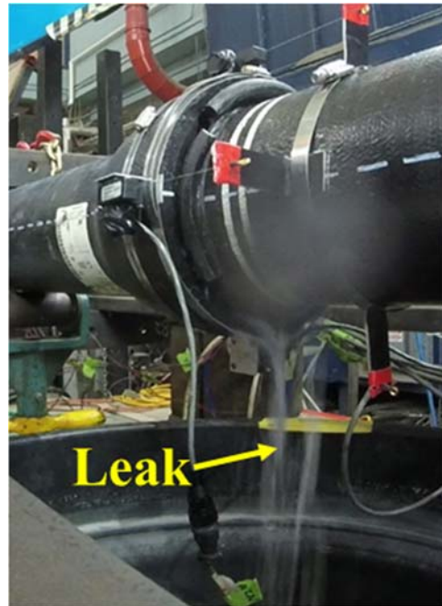
d) Pipe Leaked
