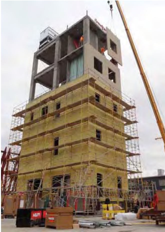
Structural skeleton during façade installation at UCSD shake table.
