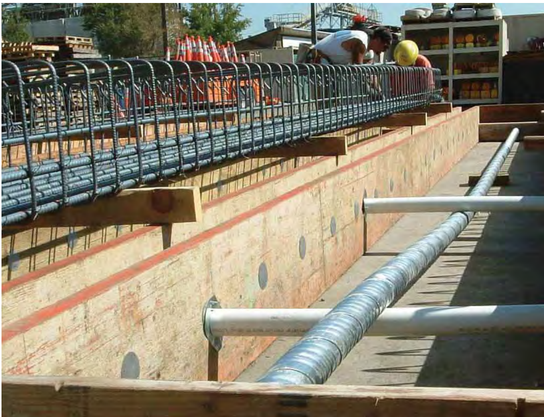
Checking longitudinal post-tension duct path prior to placement of reinforcement cages.
