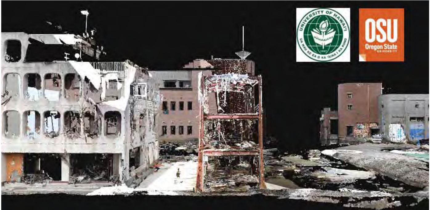
Combined LIDAR scans of buildings damaged by the tsunami in Onagawa with photographic color overlain on the point cloud.
