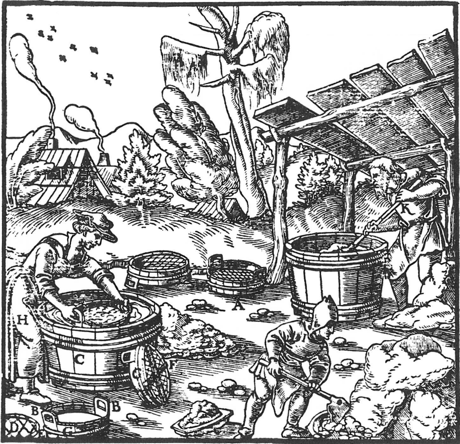
The concentration of valuable minerals as practiced during the 1500s is shown in this woodcut. Workers, including a woman on the left, are placing the ore on a screen, then jiggling the screen under water in a tub to wash away the undesirable “gangue,” leaving the desired ore. The process is directly comparable to modern jigging methods. (Reproduced with permission from De Re Metallica, published by Dover Publications, Inc., New York, N.Y., 1950)
