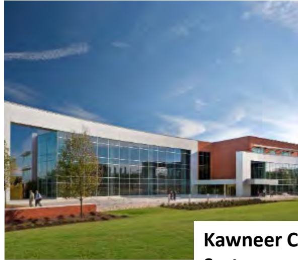
Entrances and Storefront
