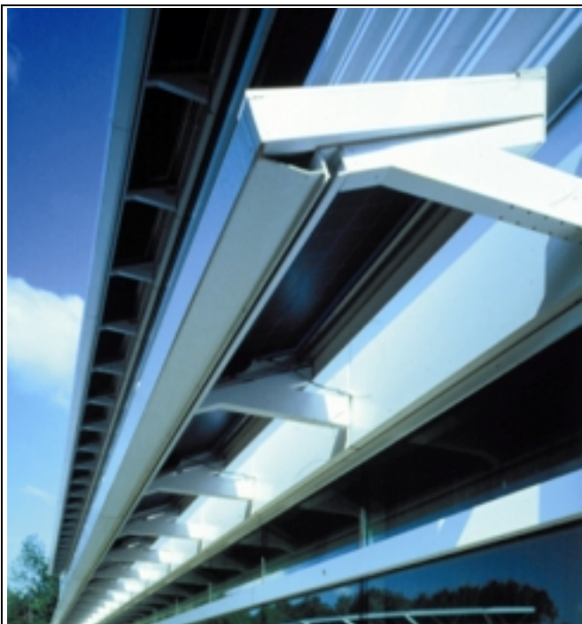
Fig. 3: BIPV sunshades in the curtainwall deliver shading and electricity at the Center for Environmental Sciences and Technology Management, at the State University of New York at Albany (SUNY) (Kawneer Company)
