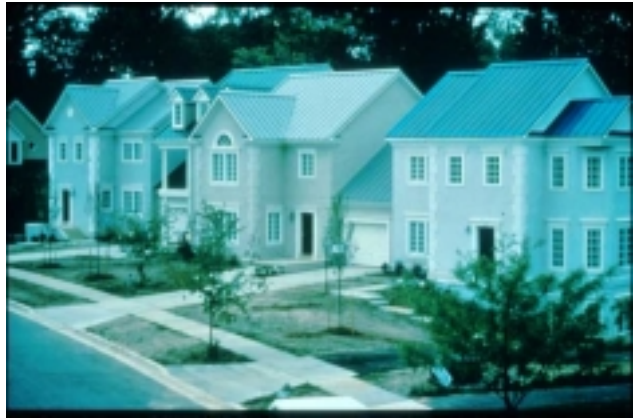
Fig. 4: Architectural standing-seam metal roof BIPV system on a townhome in Bowie, MD. (United Solar)
