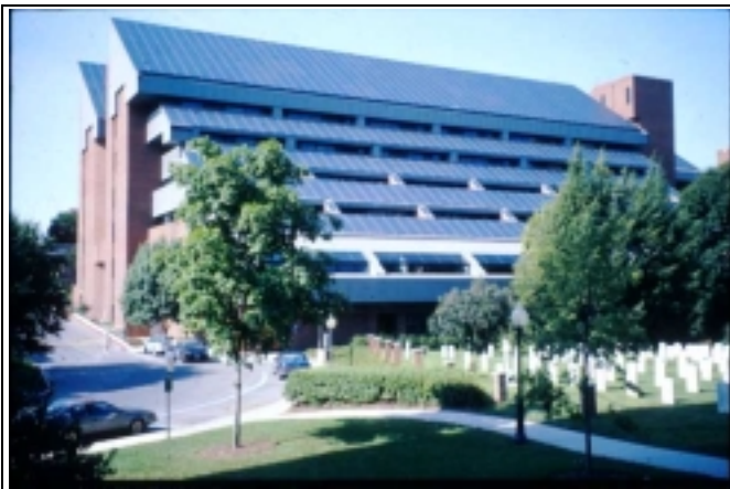
Fig. 1. The Georgetown University Intercultural Center in Washington, DC. was designed purposefully to receive a 325-kWp BIPV roof by Solarex and Kawneer. (Solar Design Associates, Inc.)
