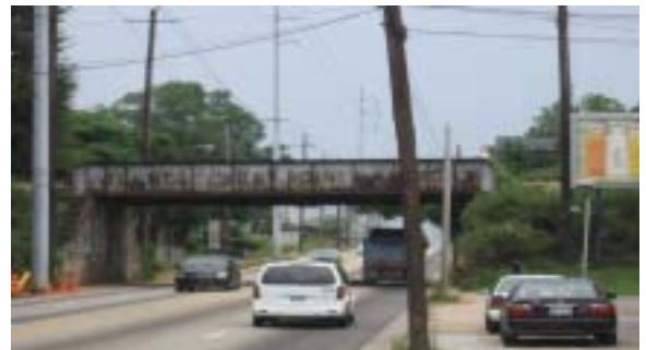
Metropolitan Parkway Overpass
