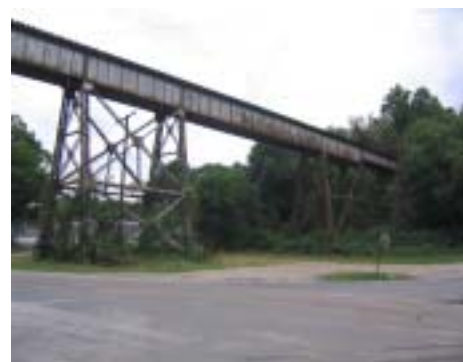
North Avenue Overpass
