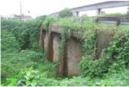
Murphy Avenue/Lee Street Overpass
