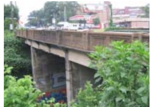
Peachtree Road Overpass
