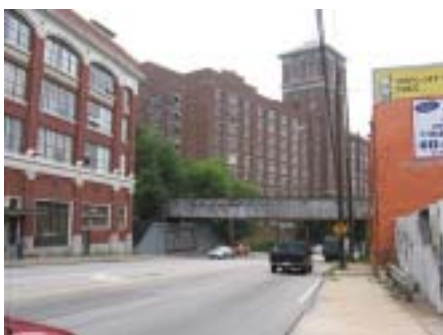
Sears Roebuck Distribution Center & City Hall East, 2005
