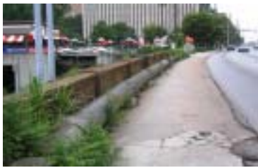
Peachtree Road overpass at CSX rail line, with 2045 Peachtree building in background
