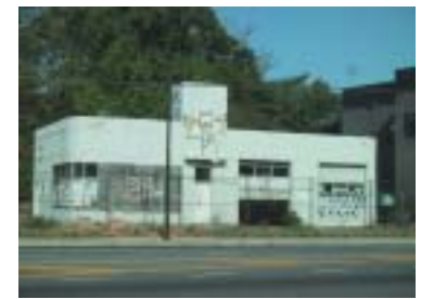
Historic filling station, 1390 Northside Drive
