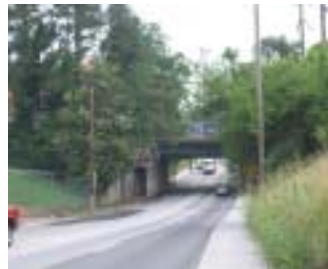
Northside Drive and 16th Street Bridge Underpass
