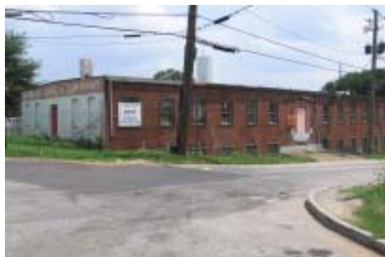
708 Jefferson Street, Guardian Chemical Company, constructed in 1890
