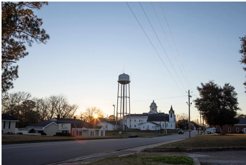
Hayneville's town square. The infrastructure package targets funding toward “disadvantaged” areas like Hayneville and surrounding towns, part of the Biden administration's goal of redressing structural racism. Charity Rachele for The New York Times
