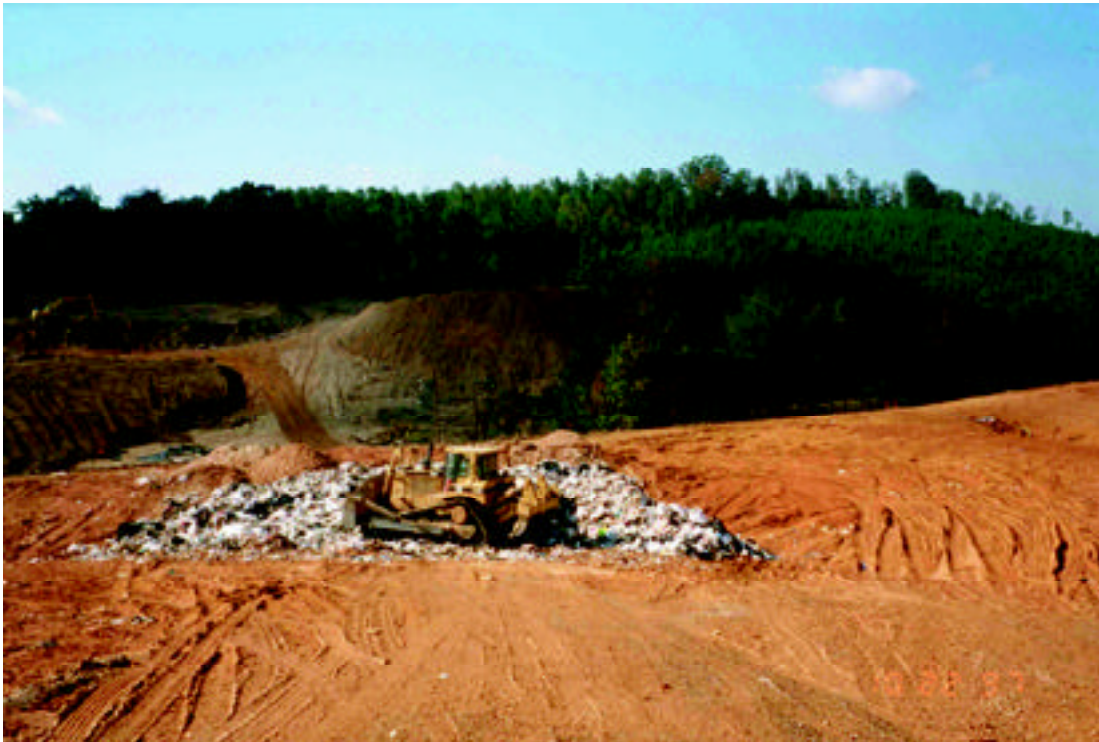
An authorized non-hazardous waste landfill
