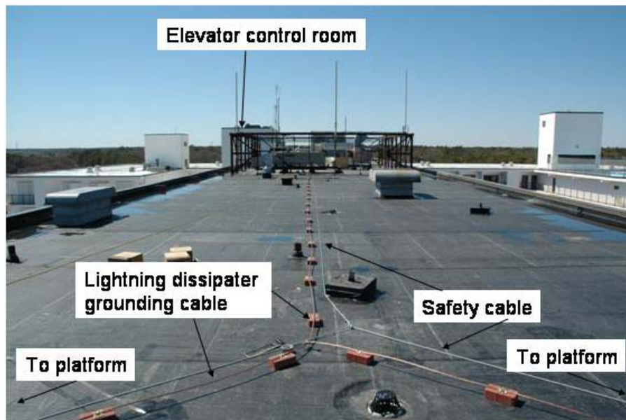
Figure 6. Image showing the grounding cable and safety cable being anchored back to I-beams located roughly halfway across the roof top.
