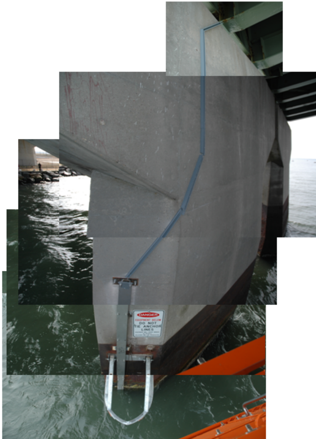
Figure 3.19: Composite of photographs taken from the UBIV of the fender and conduits ready to receive cables.
