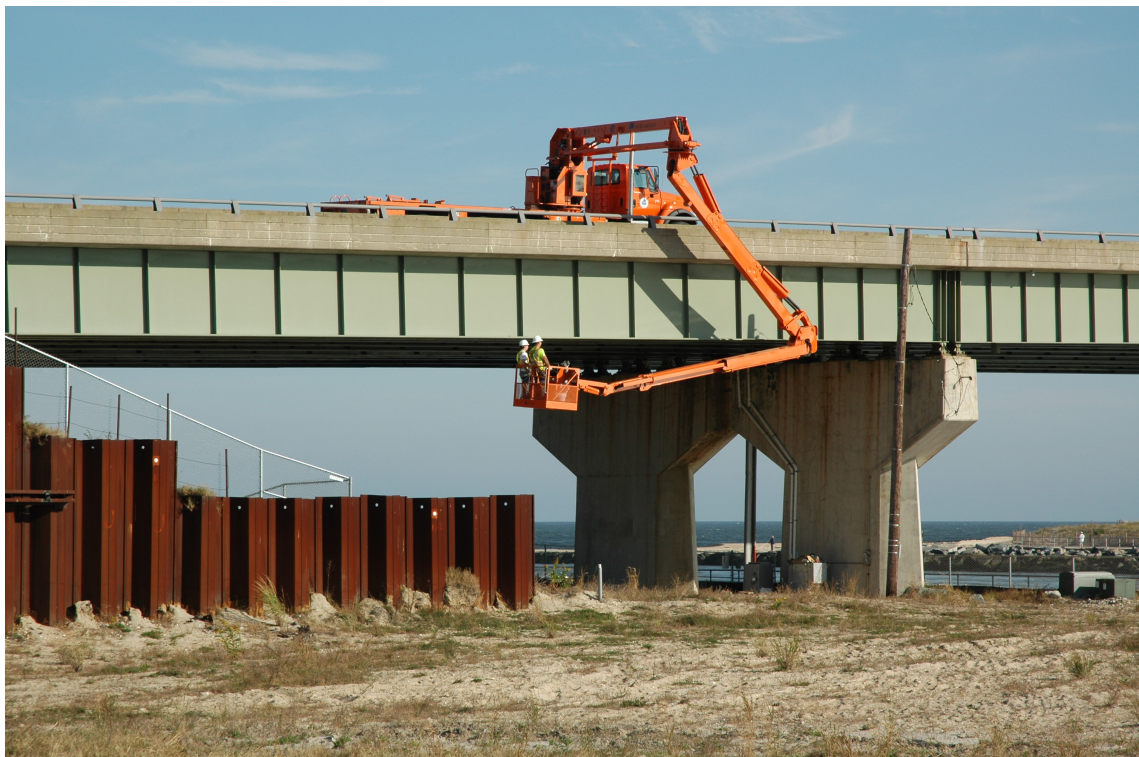
Figure 3.18: Photograph taken during Phase II that best shows the UBIV, Traffic Box, and vertical white PVC conduit on the face of the nearest pier.
