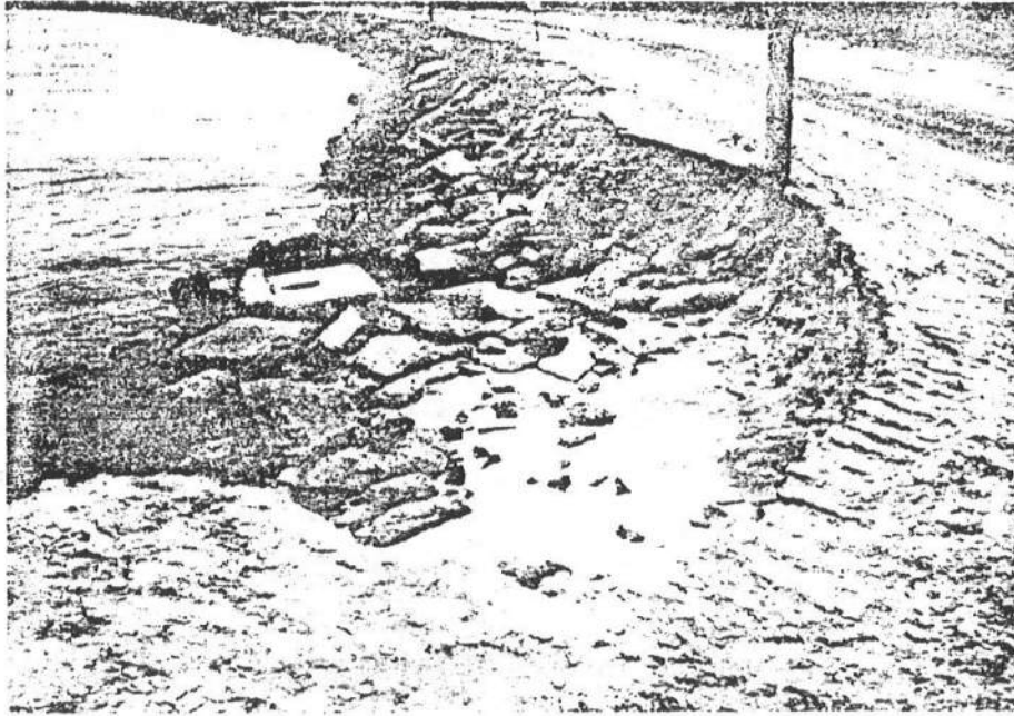
Figure 33 Breach Forming in Earthen Embankment on South Channel Bank
