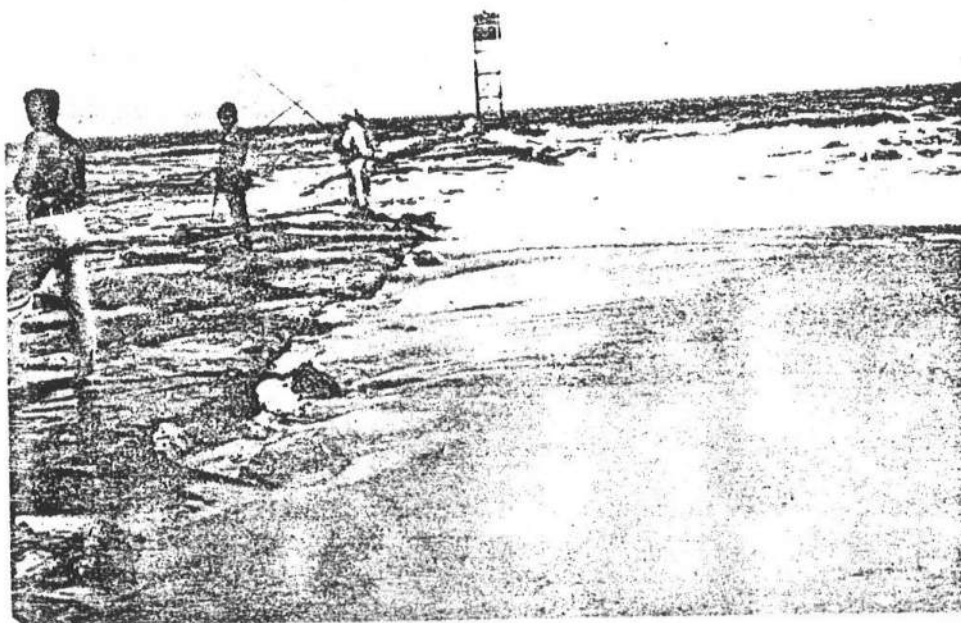
Figure 29 Sand Being Carried Over the South Jetty by Ocean Waves
