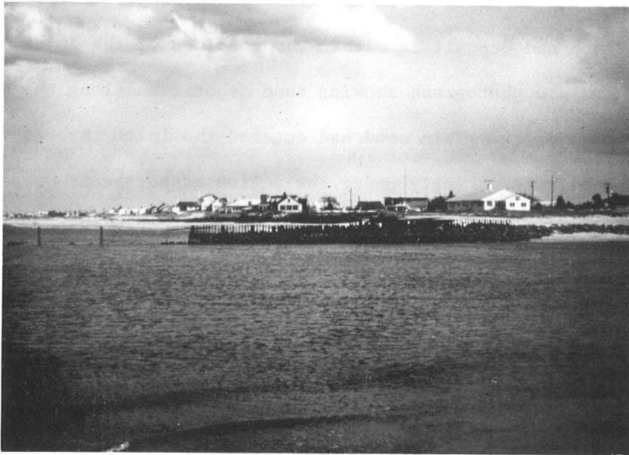
FIGURE 17 The Deposition of a Sand Mound as a Result of Over-topping the East Jetty (Right-Hand Side of Photo)
