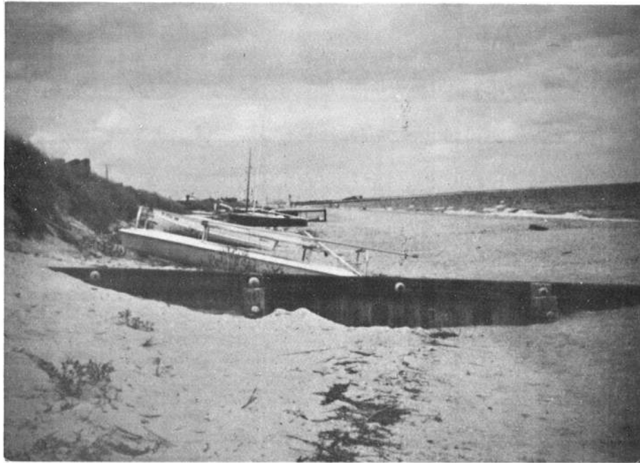
FIGURE 45 Initial Exposure of a Groin Along Lewes Beach, September, 1972 (Courtesy of Department of Natural Resources and Environmental Control, Delaware)
