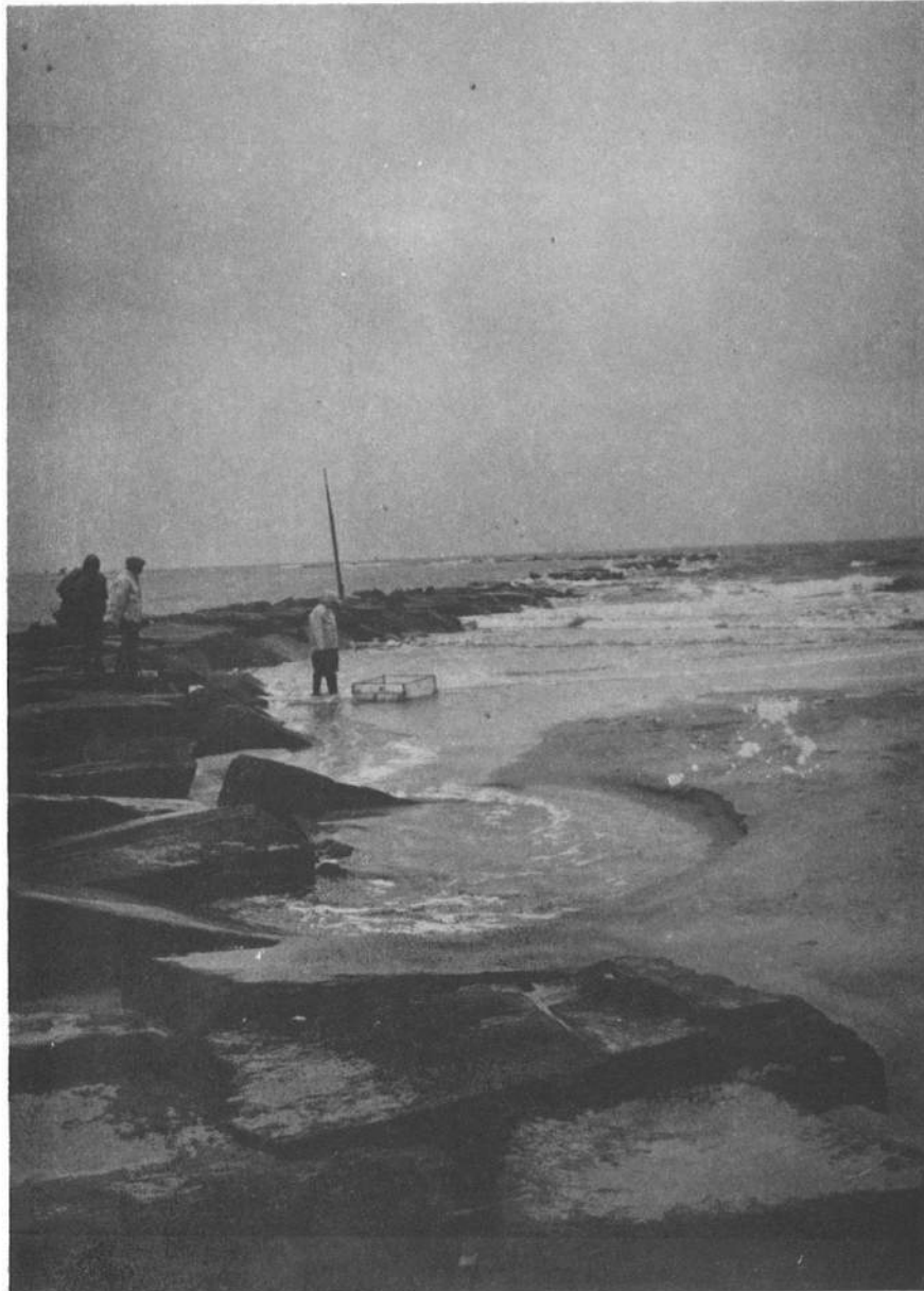
Figure 21. Photograph Showing Use of Sand Trap Looking East From South of South Jetty. Note Channel Transporting Water and Sand to and Through South Jetty.
