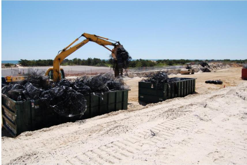
**Figure 3.4 Collection of recovered (not at Wall 1, Station 289+00) geogrid for recycling (5/23/2008).**
