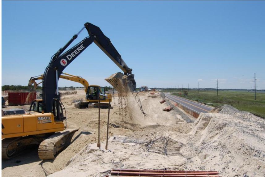
**Figure 3.2** Removal process often damaged the embedded geogrids, mainly at locations different than Wall 1, Station 289+00 (6/2/2008).
