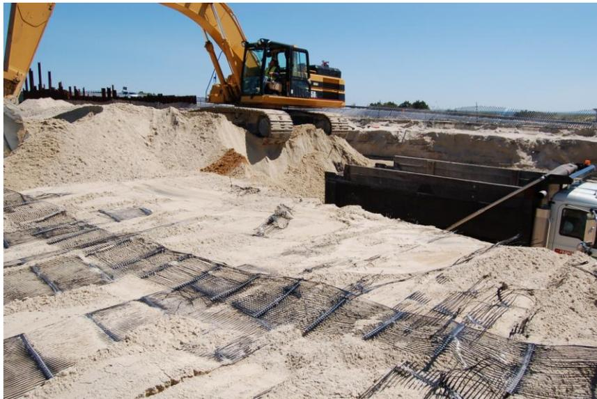
**Figure 3.3** Exposed geogrids, some damaged, and backfill loaded into a truck (6/2/2008).
