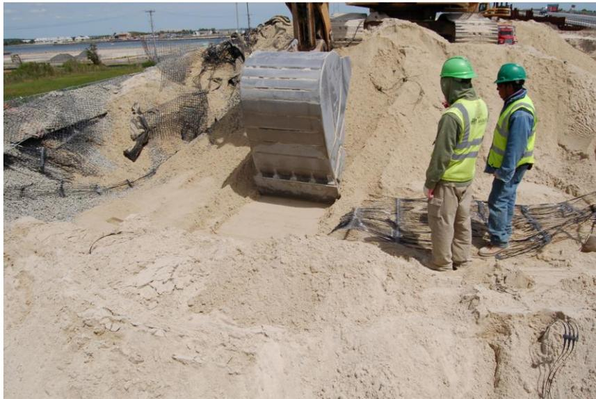
**Figure 3.5 Mechanical removal of approximately 0.38 m (15 inches) sand cover below the previous geogrid layer (5/28/2008).**
