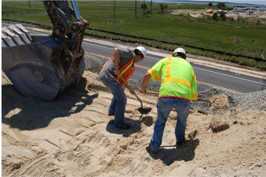
**Figure 3.6** Manual removal of the remaining 0.06 m (3 inches) of soil cover (5/28/2008).
