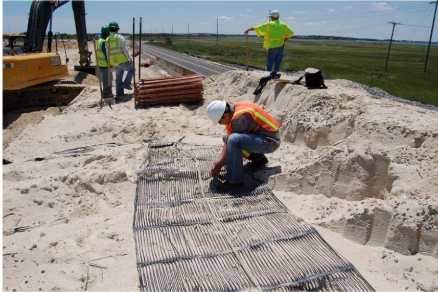
**Figure 3.8** Labeling a recovered strain gage instrumented geogrid panel (5/28/2008).
