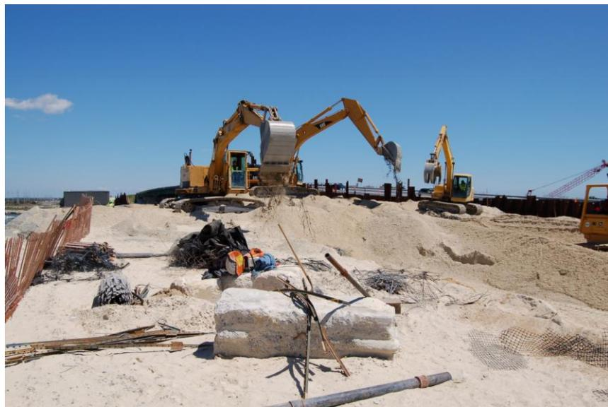
**Figure 3.1** Removal process of backfill (5/23/2008).
