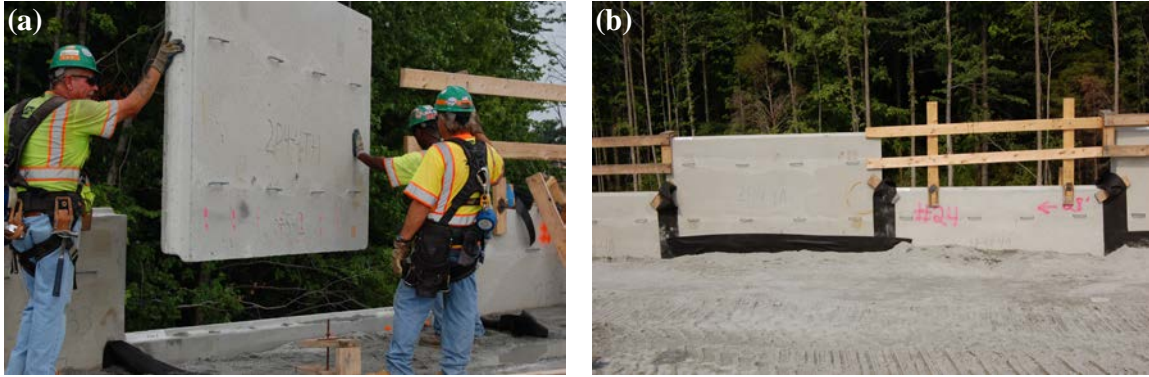
FIGURE 3 Standard precast concrete panels at the instrumented section.
