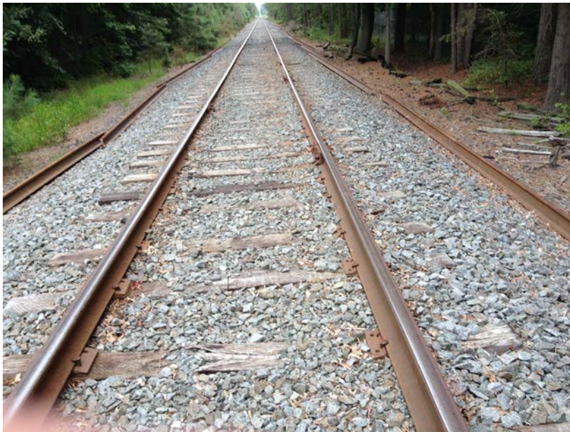
Figure 13: Delaware Coast Line Track near Airport Industrial park with new 132 RE rail awaiting installation.
