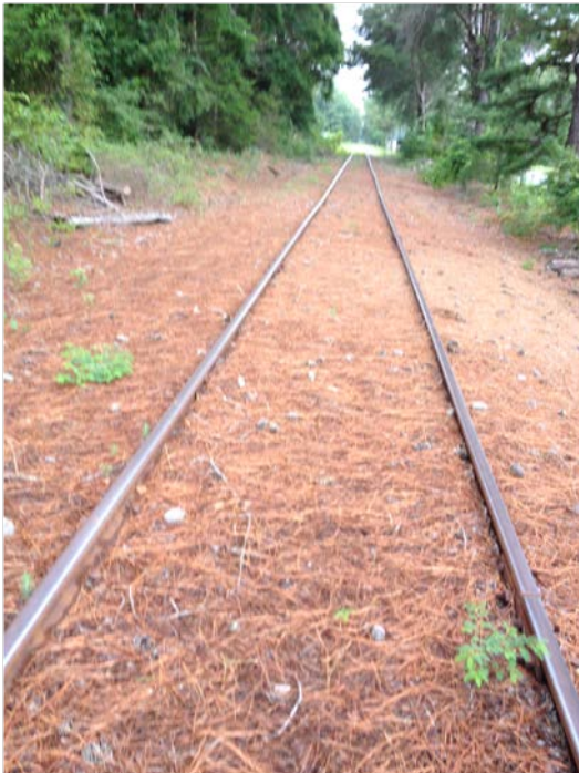
Figure 16: Segment of Milton- Ellendale line covered with Pine Needles
