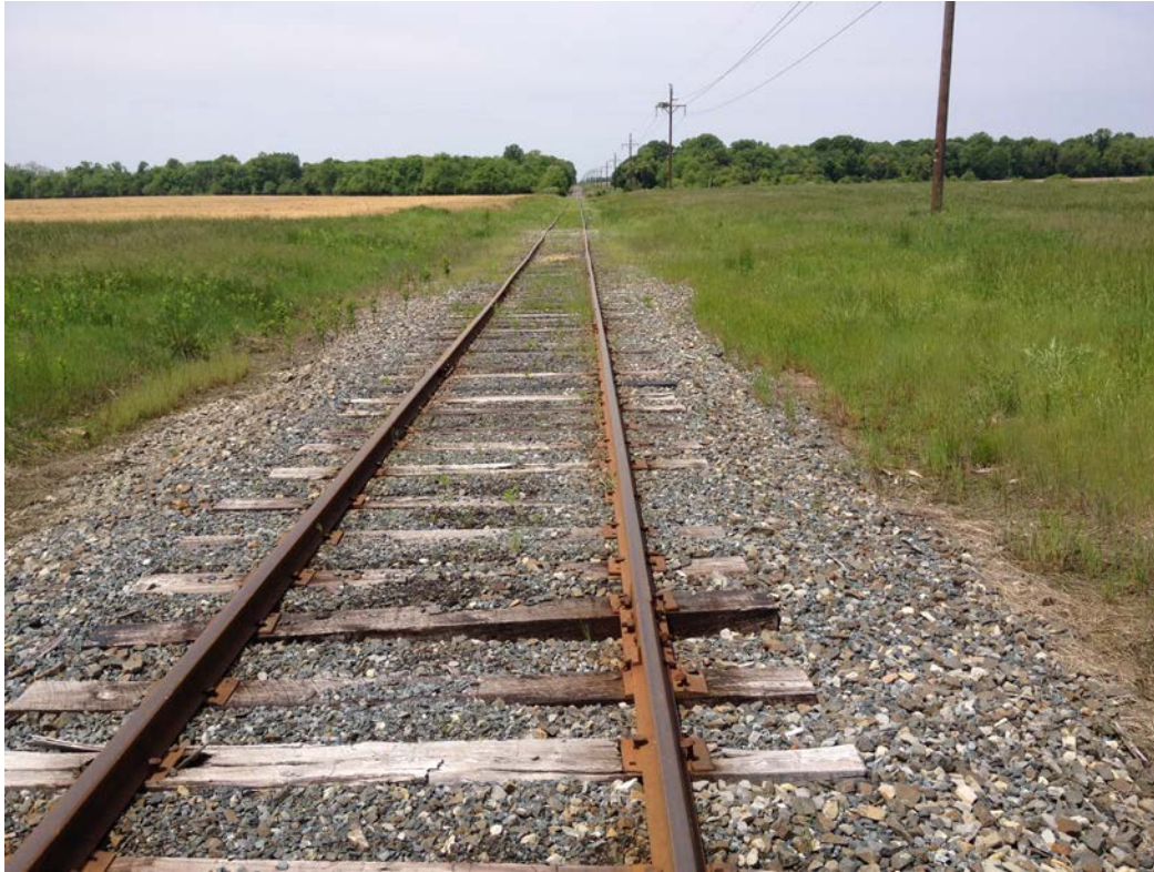
Figure 1: Overview of short line track condition
