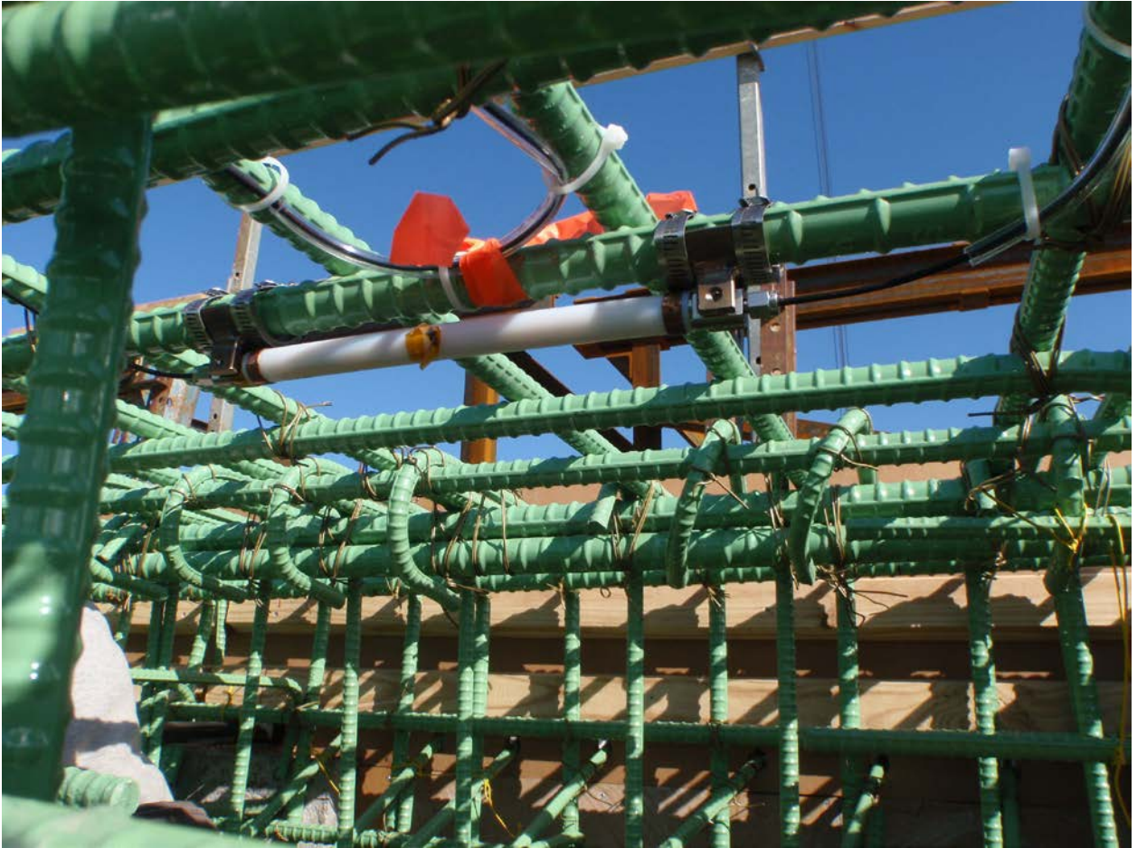
Figure 3.9. Photograph showing strain sensor installed at top of edge girder
