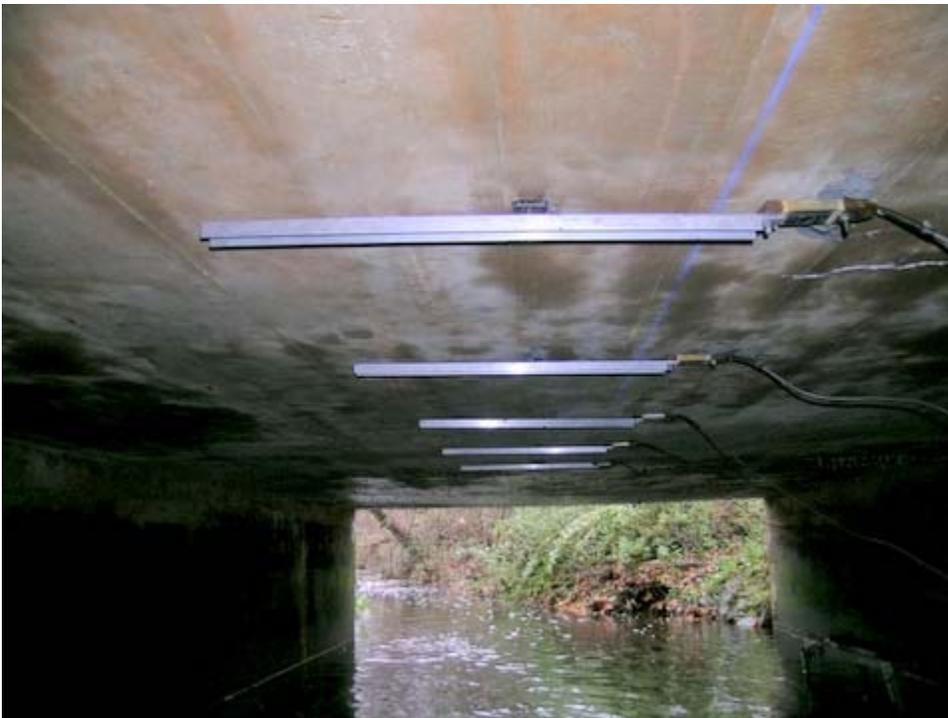
**Figure 4. Strain Transducers Mounted to Bridge 1-442 (Old Section)**
