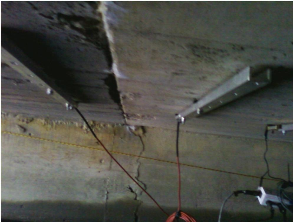
Figure 4. Longitudinal joint and adjacent sensors
