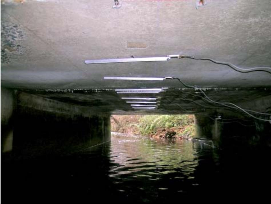
**Figure 3. Strain Transducers Mounted to Bridge 1-442 (New Section)**
