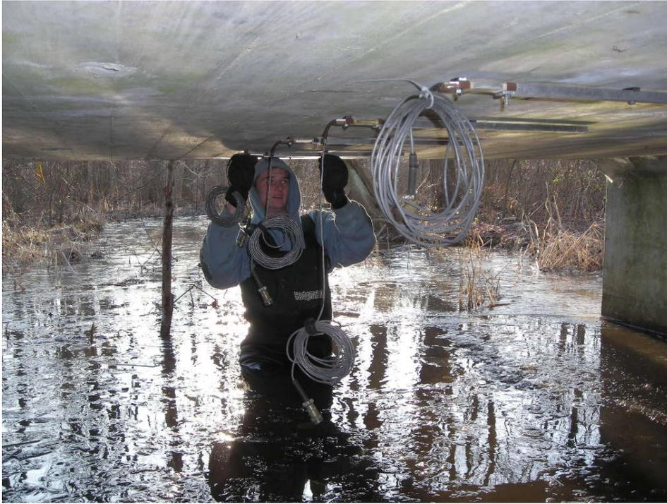
Figure 3. Mounting transducers
