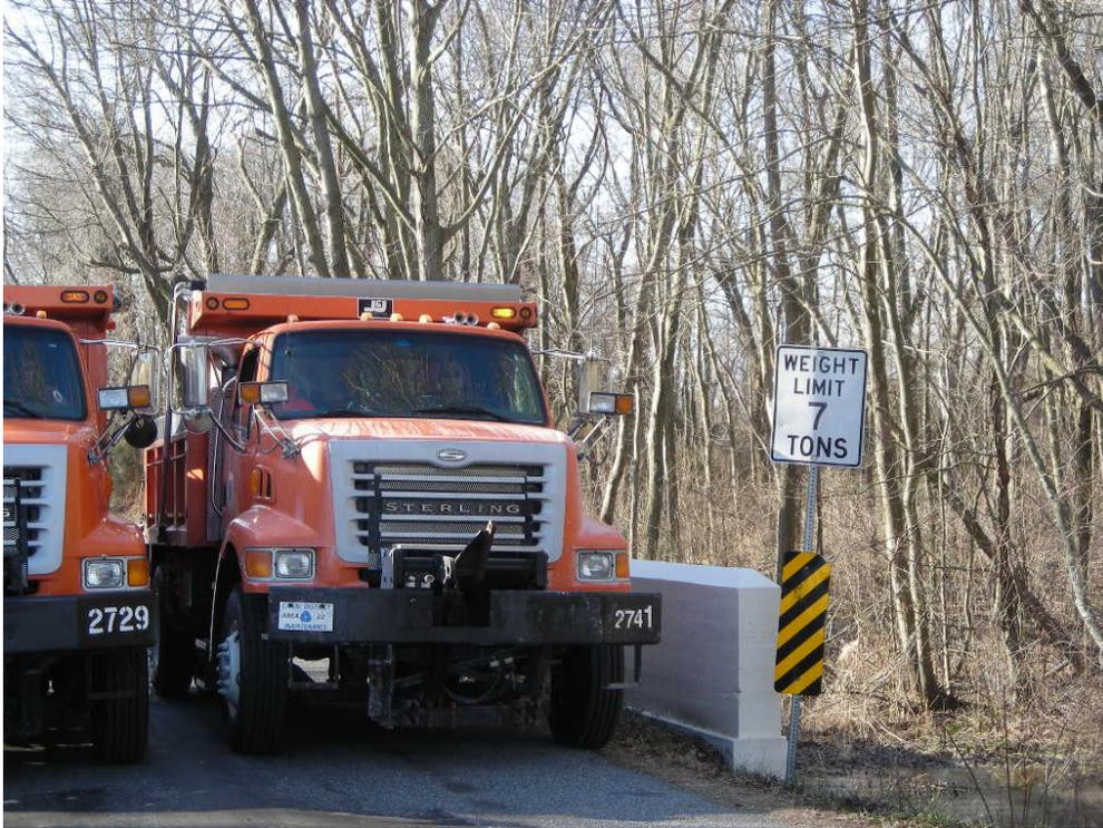
Figure 12. Trucks #2729 and #2741 (36 ton combined load) on 7 ton posted bridge
