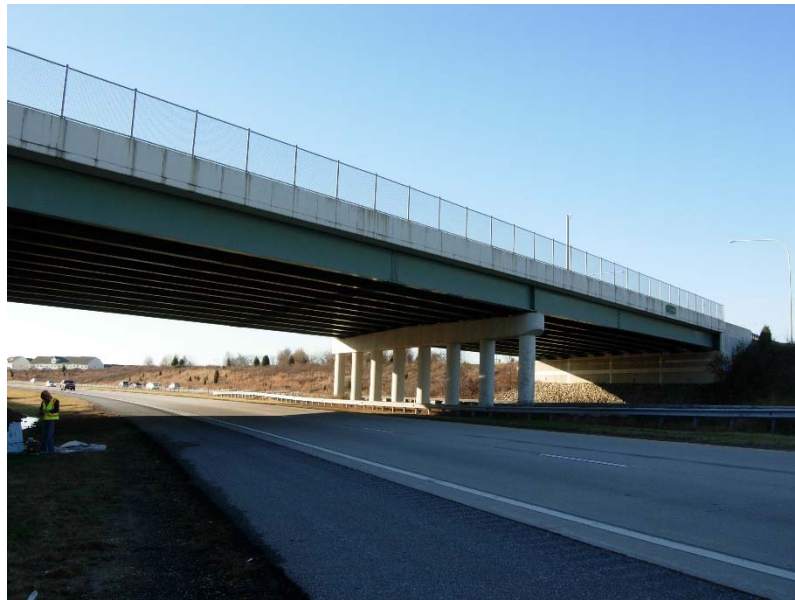
Figure 2.10 Photograph of SR 299 Over SR 1, Elevation View
