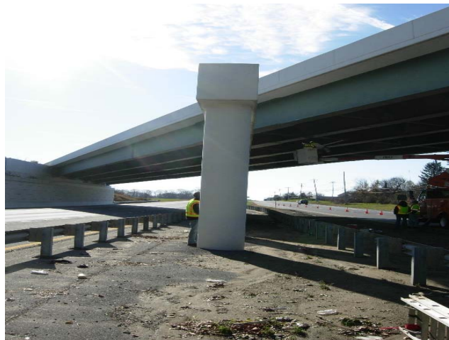
Figure 2.2 Photograph of SR 1 Over US 13, Elevation View
