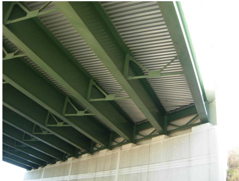
Figure 2.16 Photograph of SR 299 Over SR 1 Cross-frames
