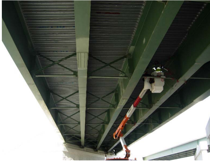
Figure 2.8 Photograph of SR 1 Over US 13 Cross-frames
