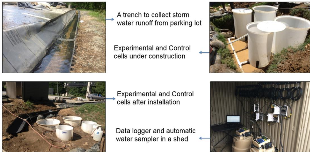
Figure 2. Photos of field construction and instrumentation of pilot-scale field facility.
