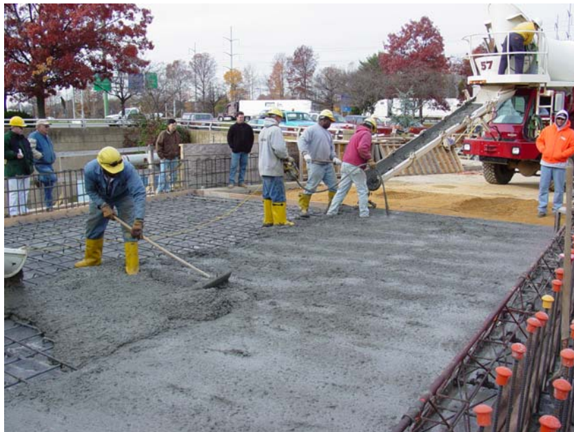
Figure 3.8 Concrete Deck Being Poured
