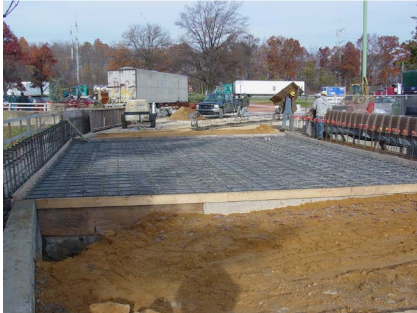
Figure 3.7 All of New Beams Placed on Bridge
