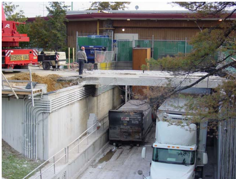
Figure 3.2 Bridge 1-712B with Old Beams Partially Removed
