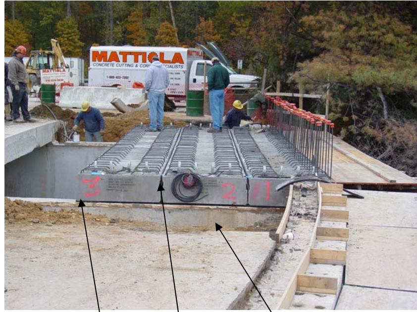
Retaining Wall Bearing Pad Grouted areas Back of
