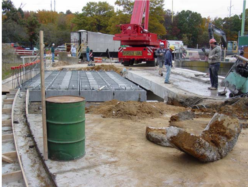
Figure 3.3 New Beams Next to Old Beams
