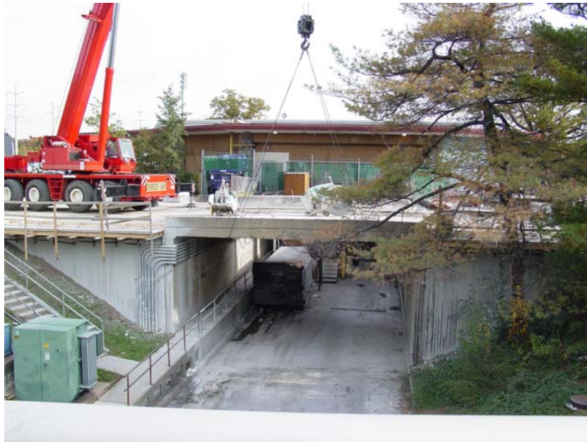
Figure 3.1 Bridge 1-712B Looking North East
