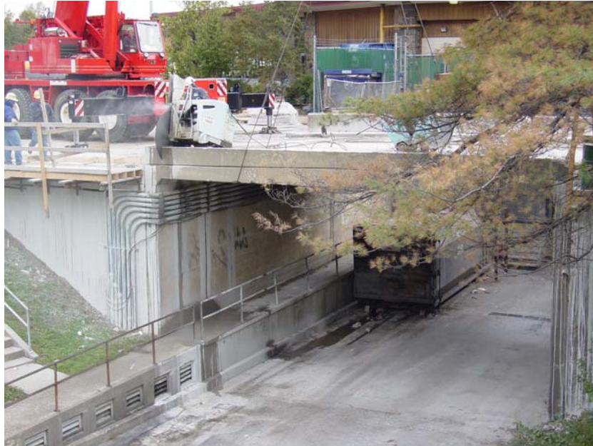
Figure 3.5 Saw Cutting and Removal of Old Beams
