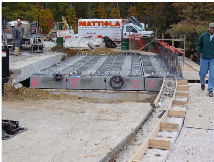
Figure 3.6 New Beams Placed on Bridge
