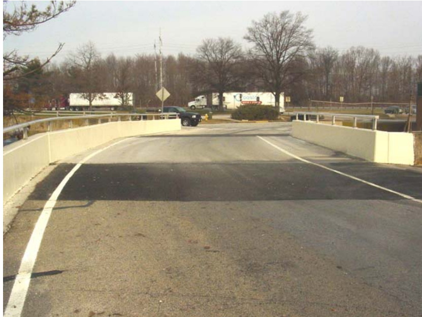
Figure 3.9 Completed Bridge 1-712B
