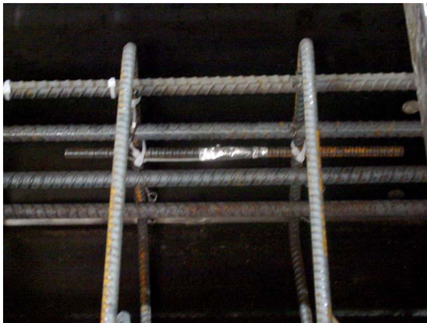
Figure 3.19 Strain Gage Attached to Bottom of Beam
