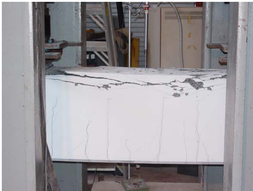
Figure 4.22 Failure of the CFRP Reinforced Beam
