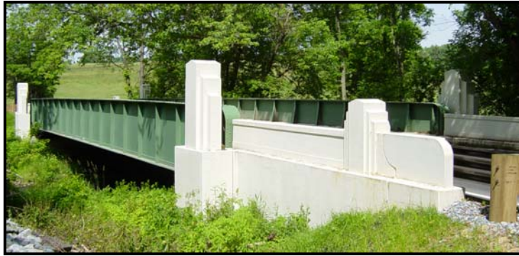
Figure 1. Ashland Bridge, looking North-West
