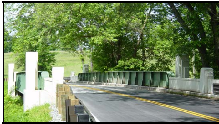
Figure 2. Ashland Bridge, looking East
