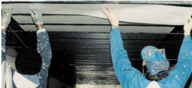
Figure 4 - Attaching composite laminates to the underside of a bridge's floor beams
