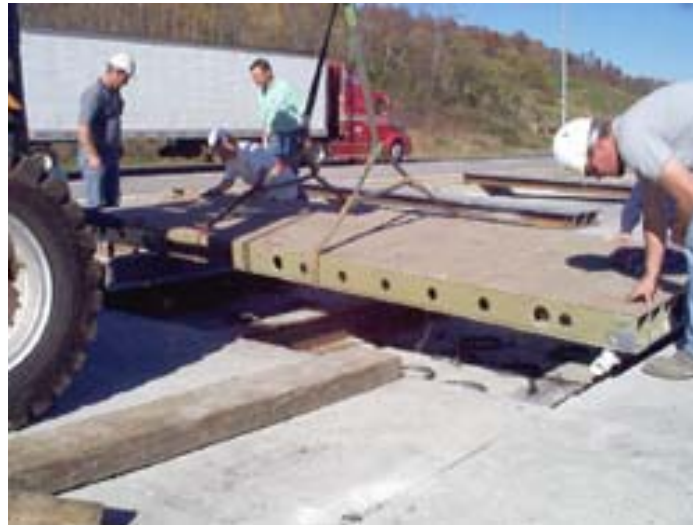
Figure 5 - Replacement of a Concrete Bridge Deck with a GFRP slab
