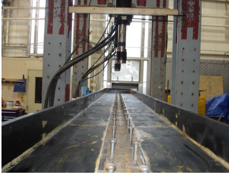
Figure 4.13 Application of Thin Oil Layer to the Wood Formwork
