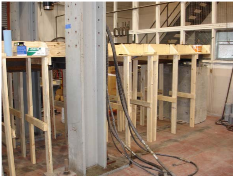
Figure 4.12 Construction of the Wood Formwork, Side View
