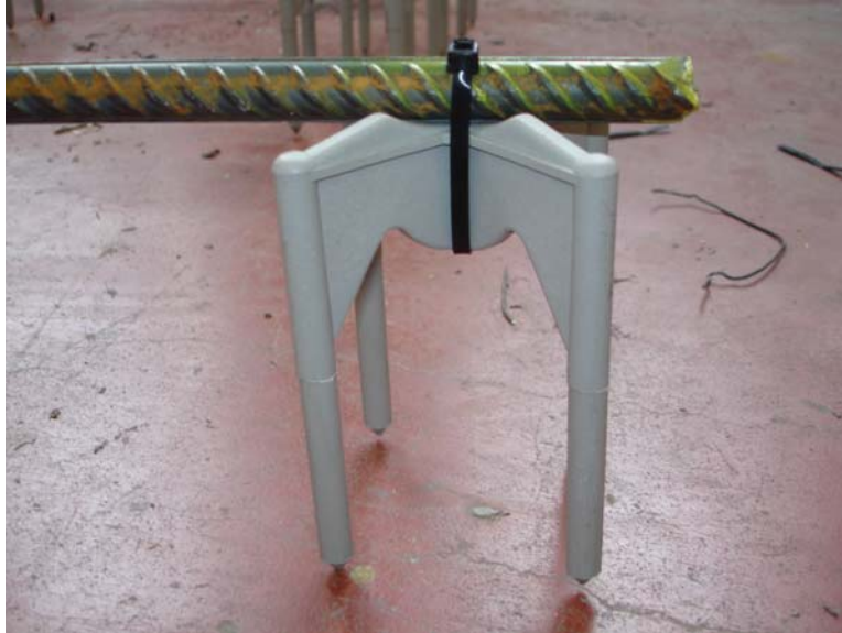
Figure 4.14 Zip Tie Connection of the Plastic Chair to Reinforcement Steel
