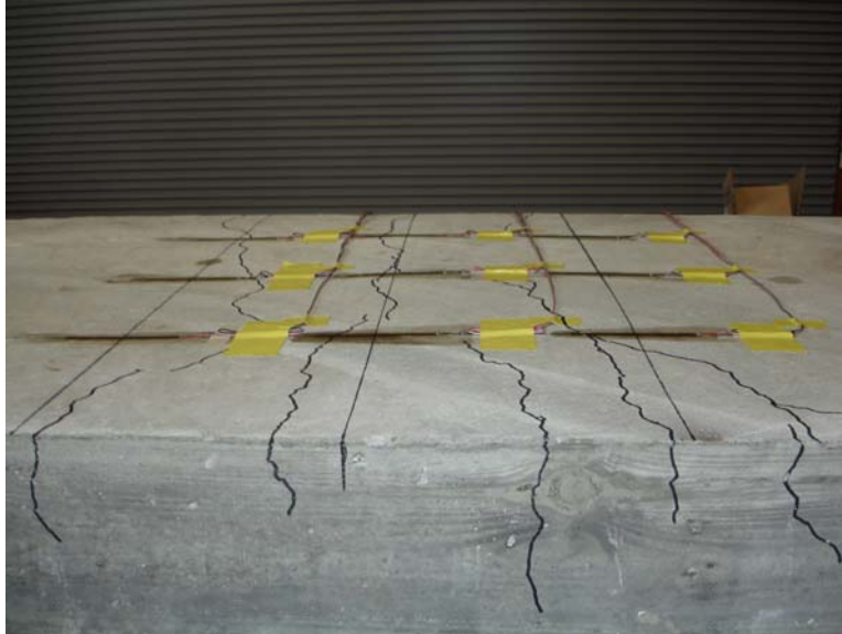
Figure 4.26 Continued Cracking throughout the Interior Pier Concrete Slab Region during Deflection Step 3
