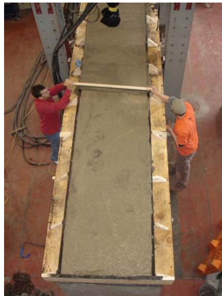
Figure 4.18 Leveling of the Poured Concrete
