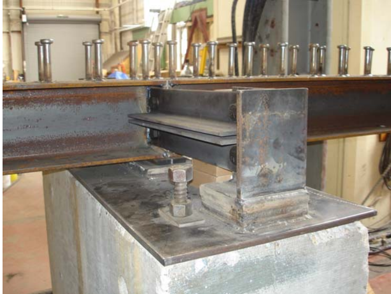
Figure 3.12 Lateral Bracing at the Interior Pier, North View
