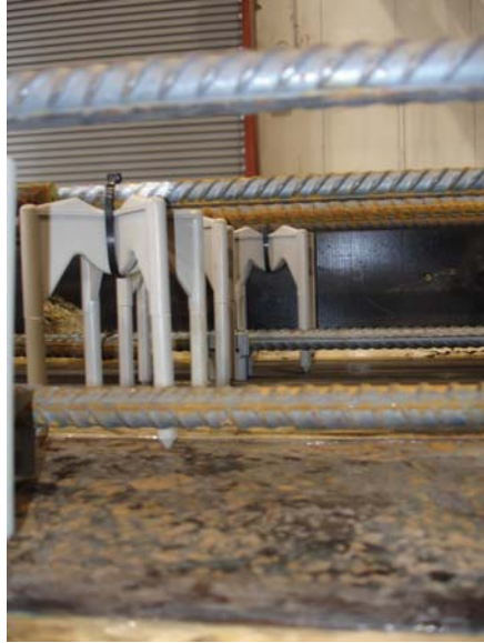
Figure 4.16 Vertical Layout of Reinforcement Steel
