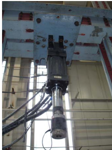
Figure 4.2 West Load Actuator in a Fully Extended Position
