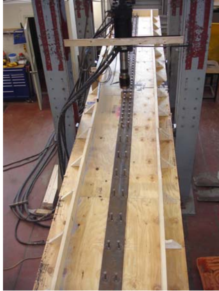
Figure 4.11 Construction of the Wood Formwork, Top View
