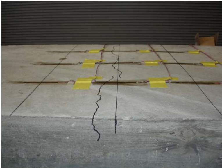
Figure 4.25 Initial Cracking through the Transverse Centerline of the Concrete Slab during Deflection Step 2
