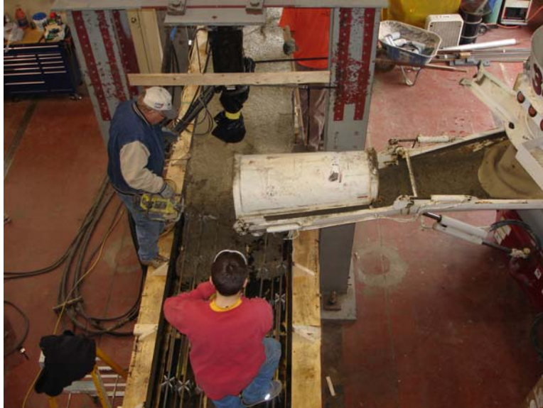
Figure 4.17 Placement and Vibrating of the Concrete
