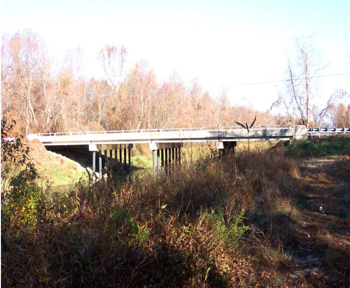
Figure 5.1 Bridge 2-063, Kent County, Delaware
