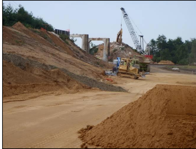
Figure 4.4 Middletown Construction Site
