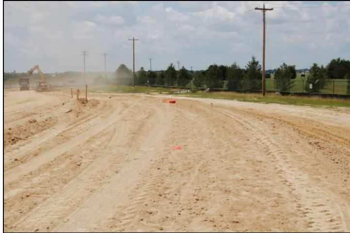
Figure 4.1 Dover Construction Site
