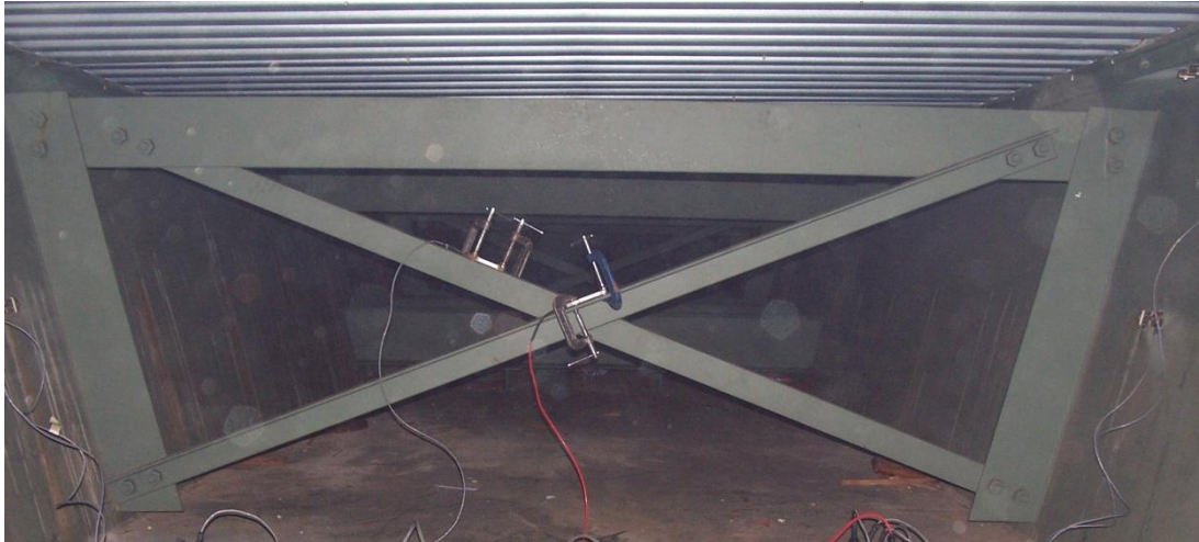
Figure 1.5 Photograph of a Type E diaphragm
