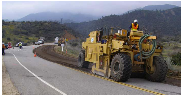
Fig. 2. Pulverizer (Flexible Pavement Rehabilitation Using Pulverization, CDOT 2008)
