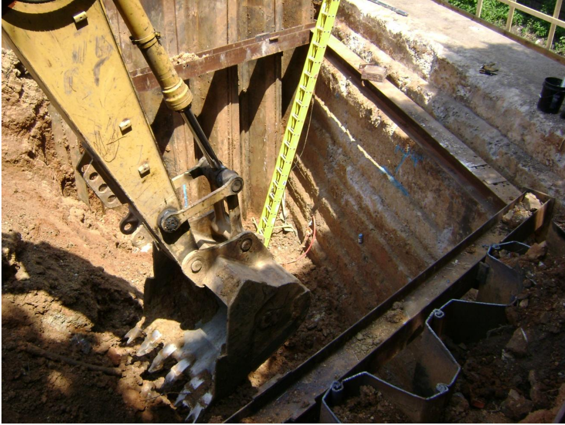
Figure 5.2 Excavation of Rear Face of North Abutment
