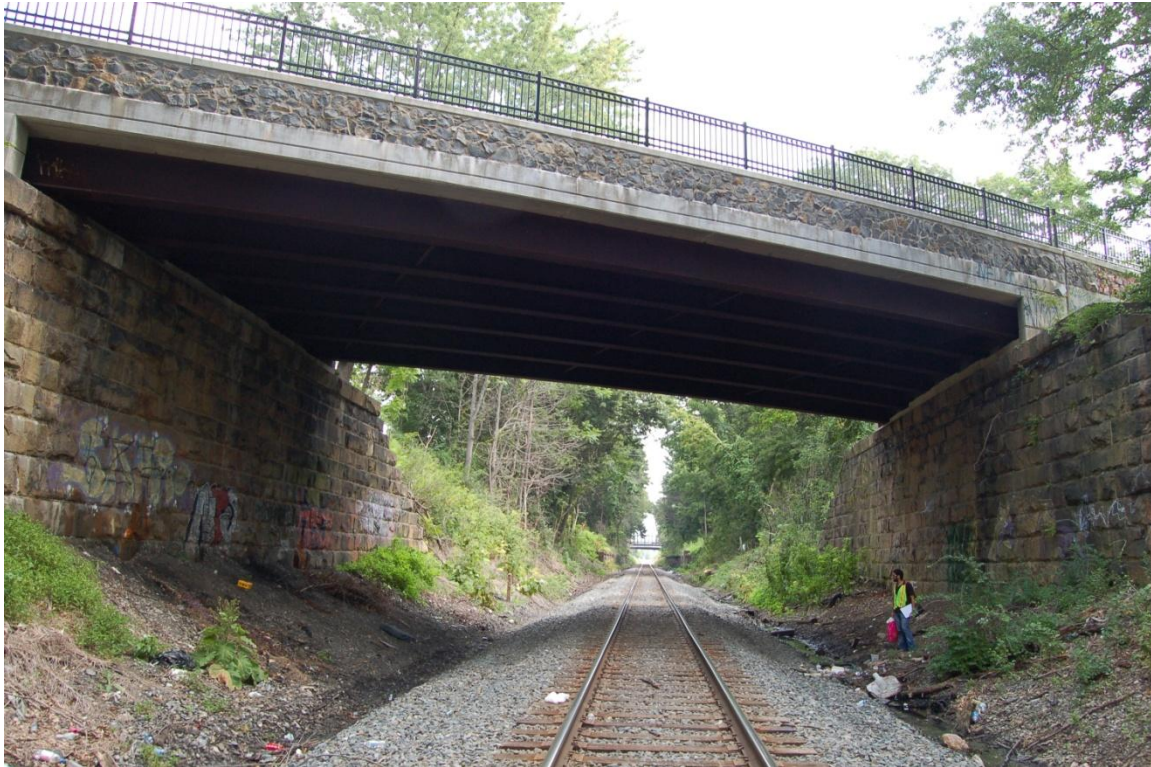
Figure 5.1 Picture of Bridge 1-609M in 2010.
