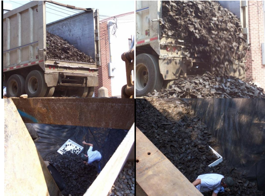
Figure 8.3. Placement of tire shreds on top of a leachate collection basin.
