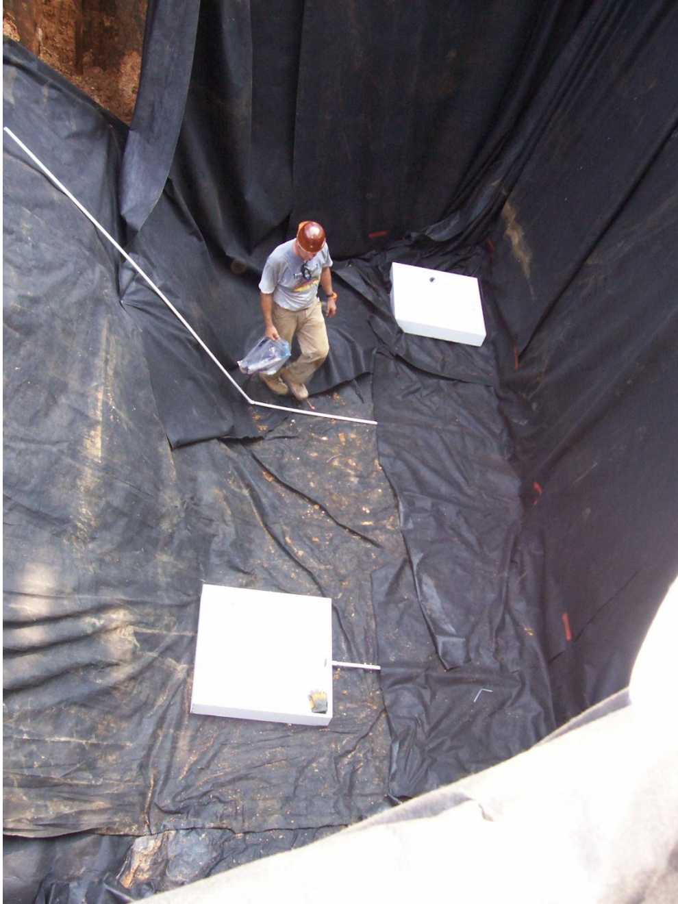
Figure 5.3 Polymeric Material in Excavation
