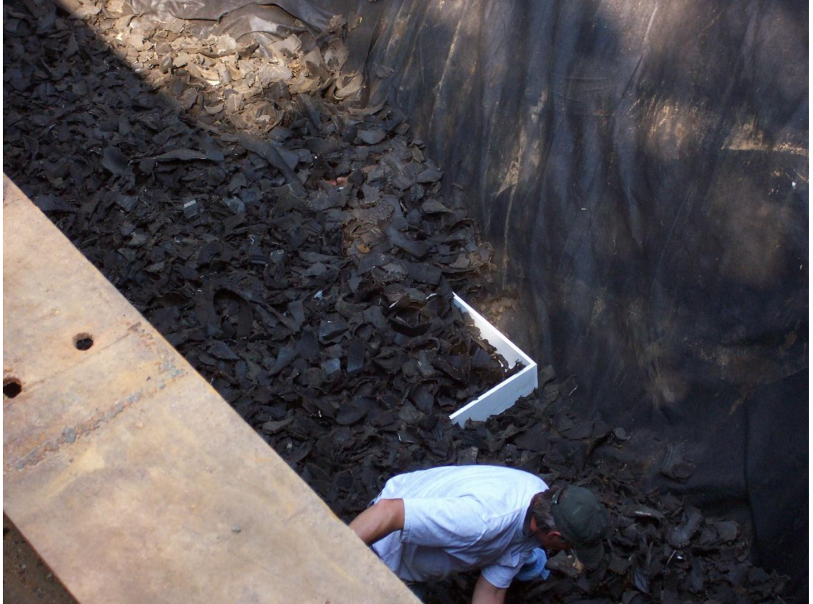
Figure 5.5 Spreading of TDA in Vicinity of Leachate Pans
