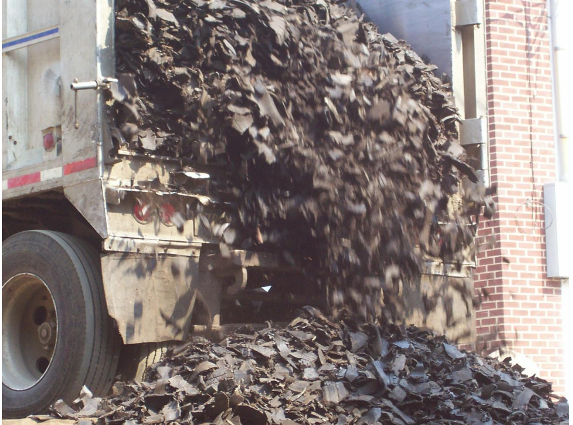
Figure 5.4 TDA is Dumped into the Excavations
