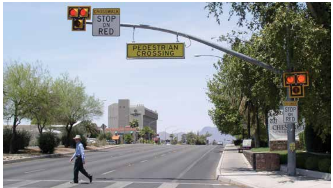
Example of a HAWK treatment in Tucson, Arizona. (Note: The pedestrian is Richard Nassi, developer of the HAWK)
