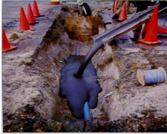
Flowable fill being placed in Fenwick Island
