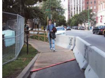
Temporary Surface Treatment
