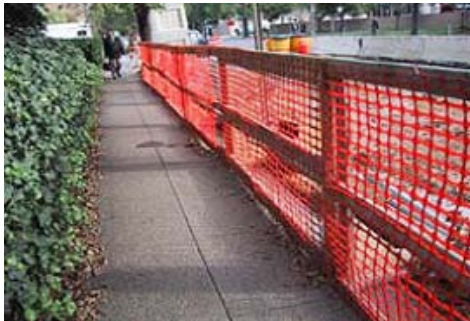
Temporary Construction Barrier Treatment
