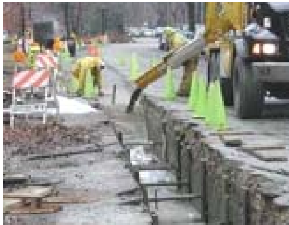
Placing of Flowable Fill
