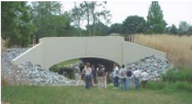
Undergraduate researchers in a summer program at the University of Delaware inspect a bridge during a tour hosted by DelDot.
