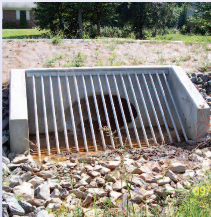
This safety grate, located in Hickory Woods in New Castle County, was one of several that were installed before fall 2004 but evaluated by Kobayashi in light of the findings in his report.
