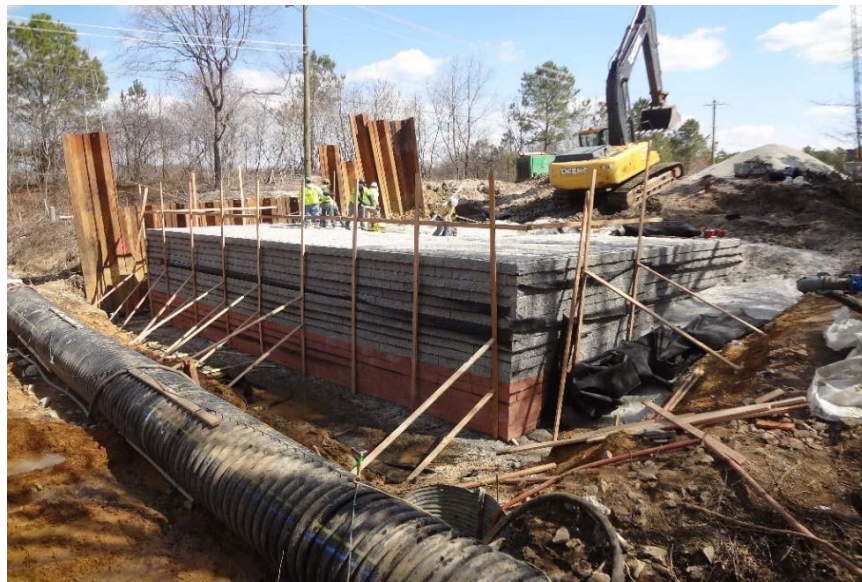
Figure 3.18 East abutment excavation and construction (4-3-13)
