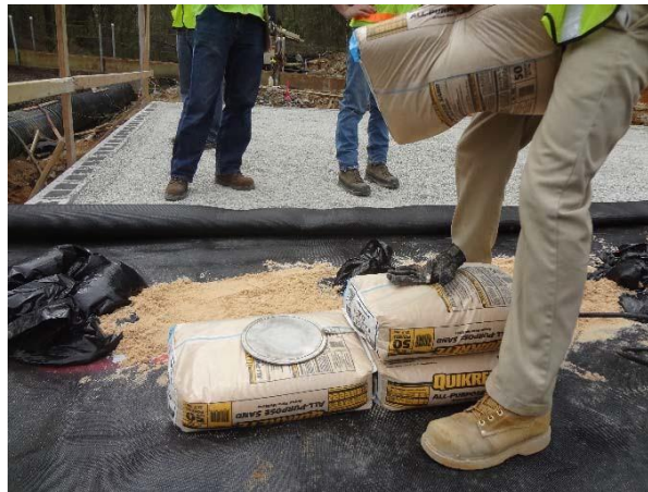
Figure 3.31 A total pressure cell and its installation
