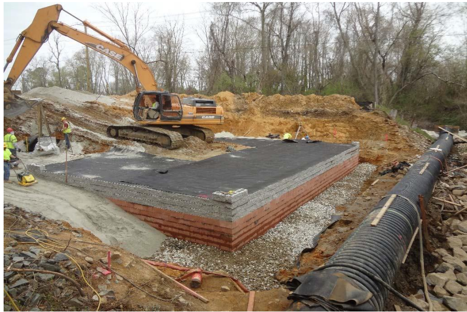
Figure 3.22 West abutment excavation and construction (4-16-13)
