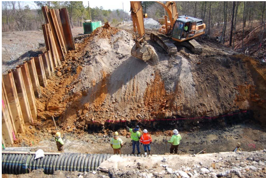
Figure 3.14 East abutment excavation and construction (3-25-13)
