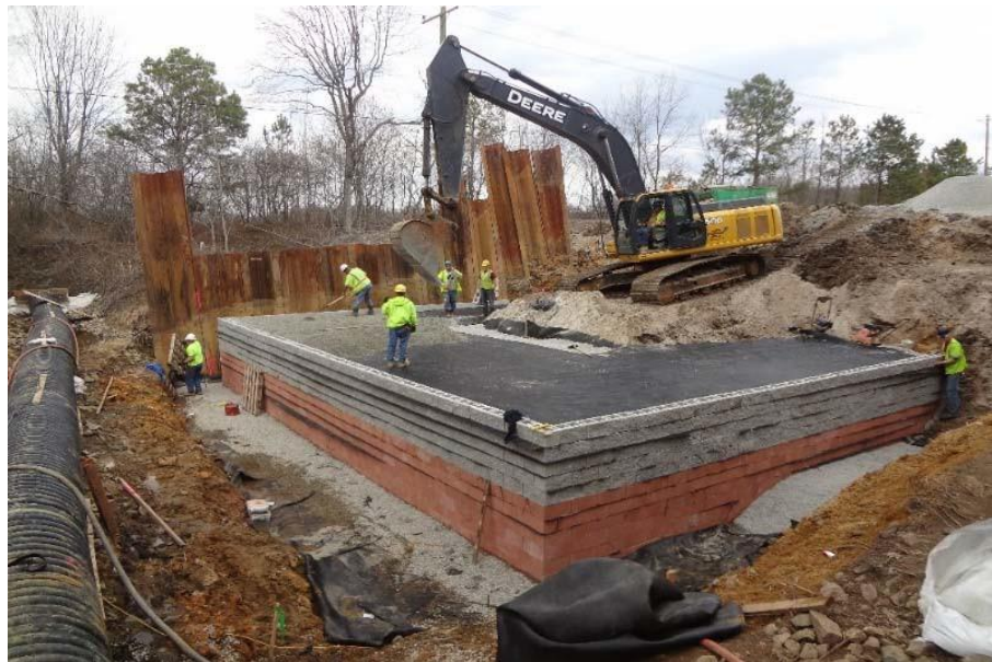
Figure 3.16 East abutment excavation and construction (4-2-13)
