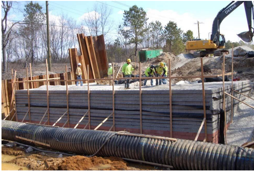
Figure 3.17 East abutment excavation and construction (4-3-13)
