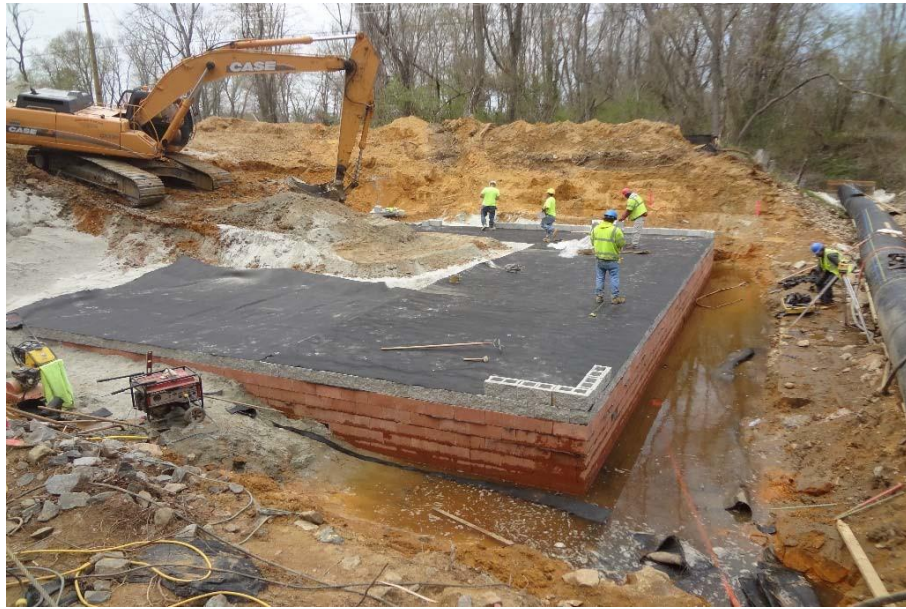
Figure 3.21 West abutment excavation and construction (4-15-13)
