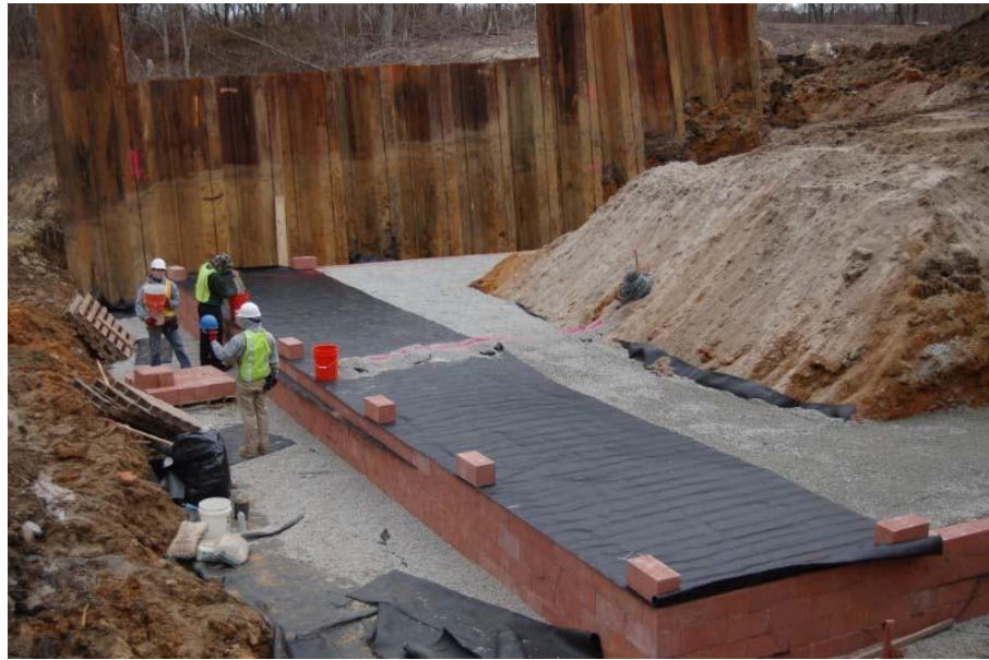
Figure 3.15 East abutment excavation and construction (3-28-13)
