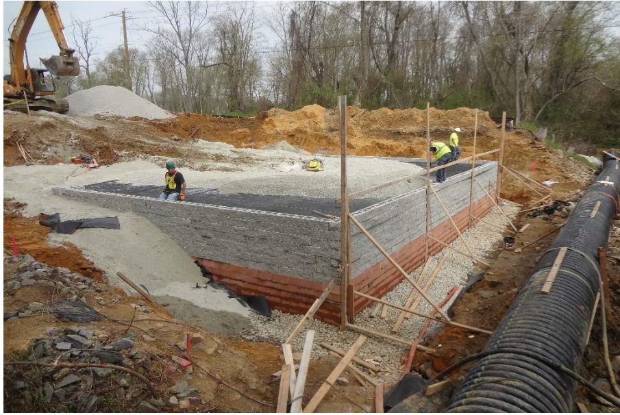
Figure 3.23 West abutment excavation and construction (4-17-13)
