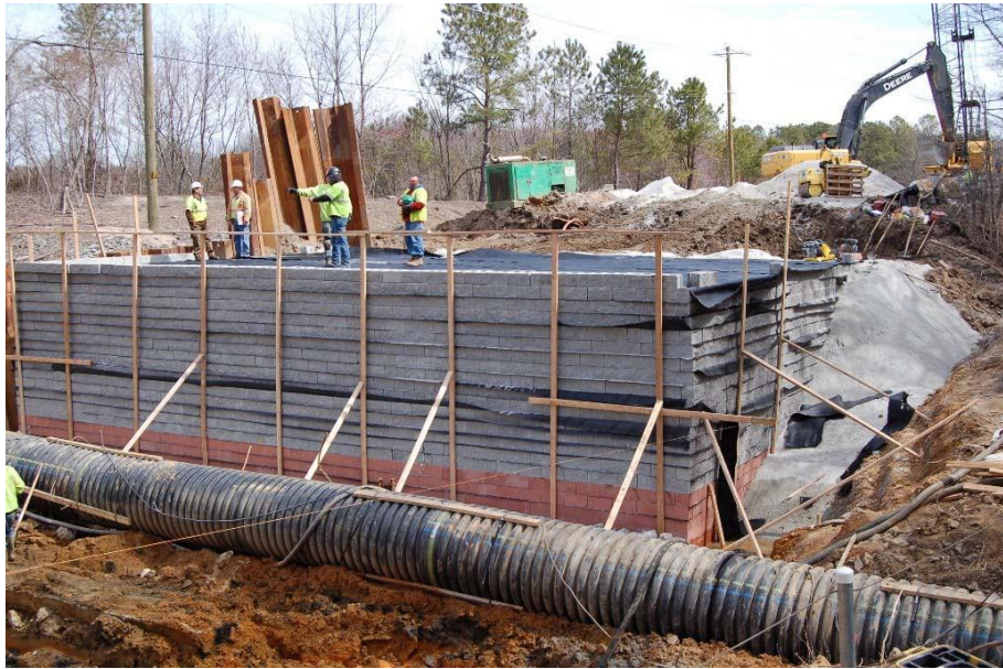
Figure 3.19 East abutment excavation and construction (4-4-13)
