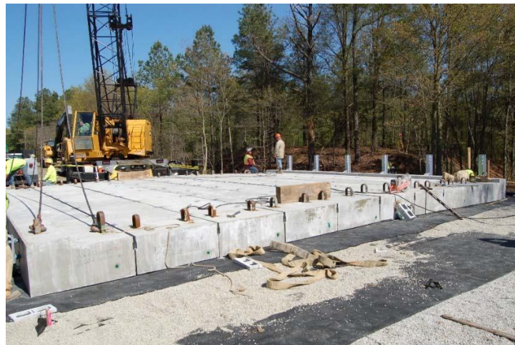
Figure 3.25 Bridge placement operation
