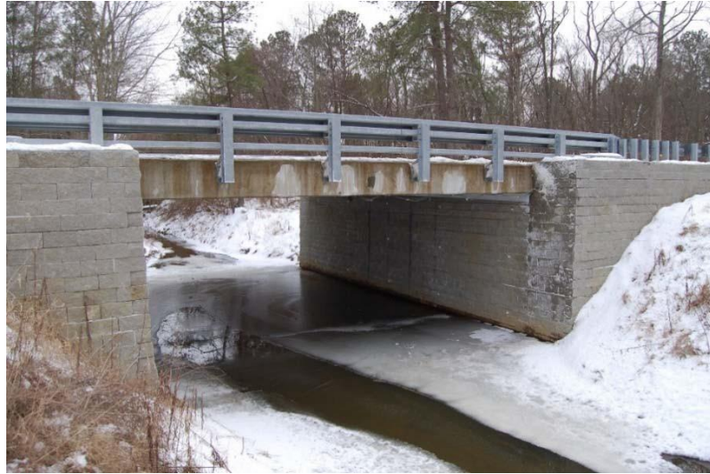
Figure 3.27 Completed bridge and abutments, eight months after construction
