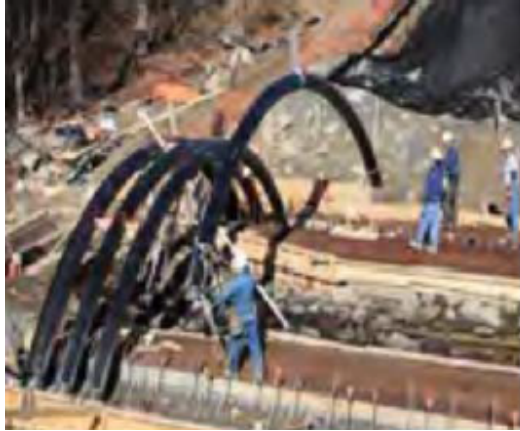
Figure 2. Photo. FRP Arches being lowered into place. Photo 6. FRP Arches being lowered into place. Reprinted from Project case studies for IBRC and IBRD Programs , D. Paterson et al., 2012, FHWA report, p.860. Unpublished internal document of FHWA.
