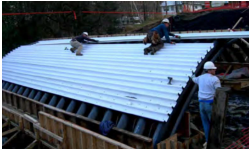
Figure 3. Photo. Sheet metal installed on FRP tubes. Photo 7. Final arch placement with corrosion resistant decking being installed. Reprinted from Project case studies for IBRC and IBRD Programs , D. Paterson et al., 2012, FHWA report, p.861. Unpublished internal document of FHWA.
