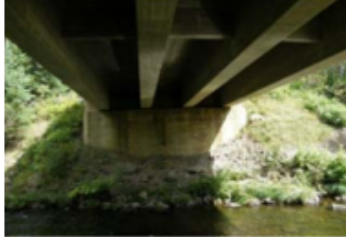
Trout Brook Bridge girders (Photograph from Bologna & Khabra (2012))
