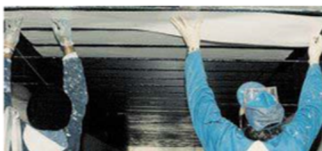
Attaching composite laminates to the underside of a bridge's floor beams.
