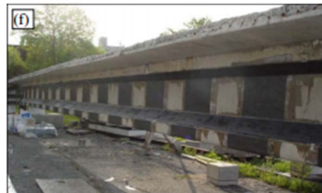
Final rehabilitated pre-stressed concrete girder with vertical CFRP strips and anchoring longitudinal CFRP strips
