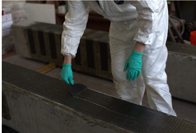
Figure 32. Smoothing the CFRP onto the surface of the beam using putty knife
