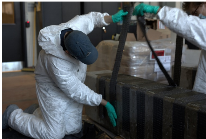
Figure 33. Installing U-Wraps onto the girder
