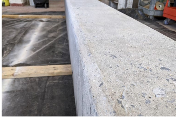
Figure 22. Typical ground edge of a girder
