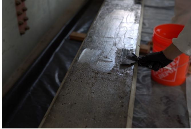
Figure 27. Applying thickened epoxy to the tensile face of the girder using a plastic putty knife
